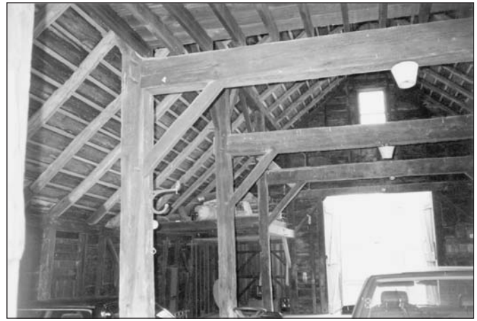
Photo 4. A second view of the Bartholf barn. The barn has an added bay at the northwest gable wall. Oak (and possibly chestnut) timbers comprise the H-frames. Anchorbeam tenons extend only about two inches with no wedges.
