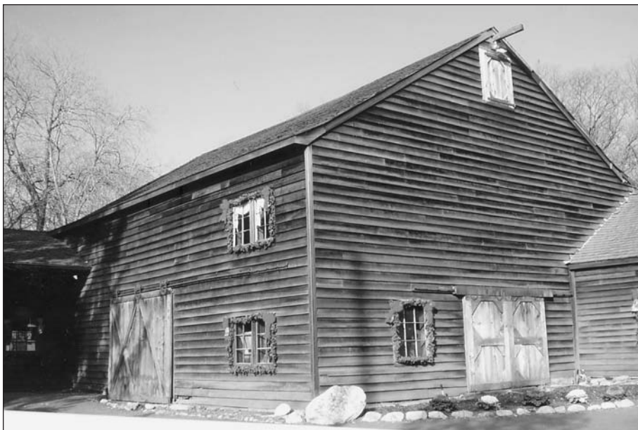
Photo 6. The extant c.1840 Yeoman-Abma three-bay converted "Dutch-Anglo" barn in Wyckoff. In its original classic form the width of the nave was 20'-6" and the original side wall length was 34 feet. Homestead is currently a fruit and vegetable farm.
