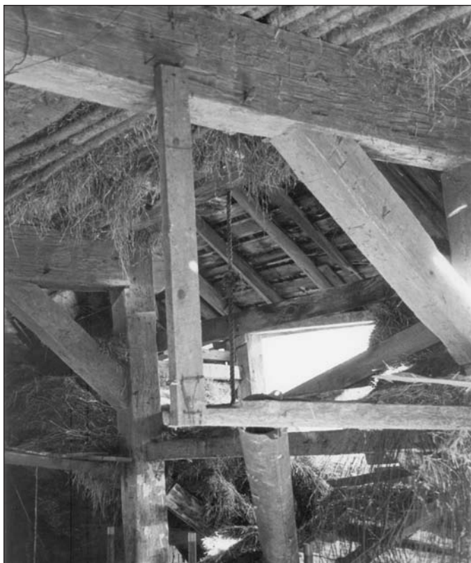
Photo 6. Interior photo showing anchor beams by Erin Willsey, 1990.
