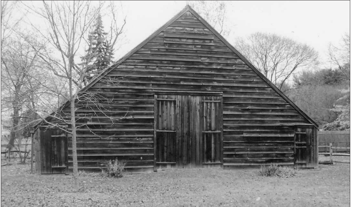
Photo 1. The extant c.1760 (dendro-dated) classic three-bay Wortendyke Dutch barn. Now a museum in Park Ridge, New Jersey, this barn features the lowest side walls—measuring six feet in height—of any known classic Dutch barn in North America. The barn measures 45 feet wide at its gable ends and 37 feet along its side walls. Many of the H-frames are comprised of tulip wood timbers.
