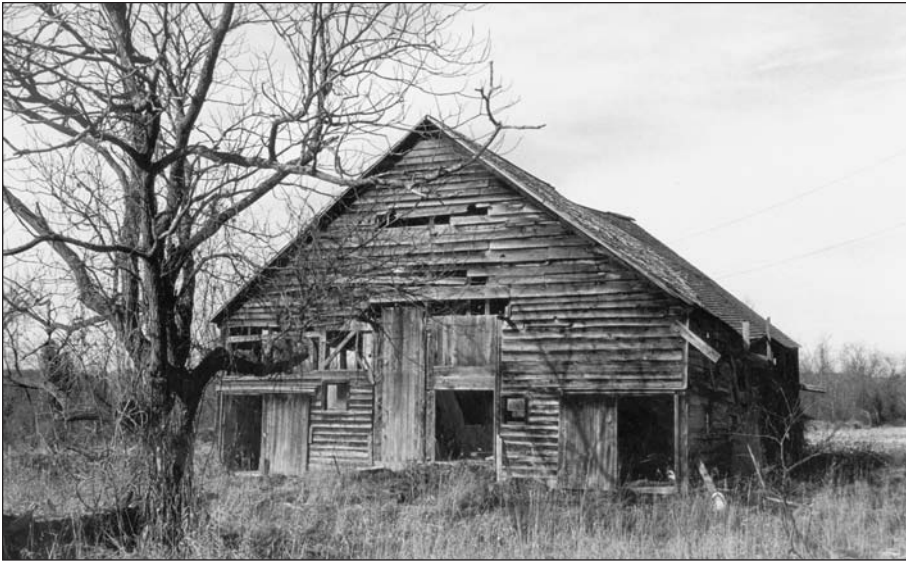
Photo 4. Exterior view of the barn by Erin Willsey, 1990.
