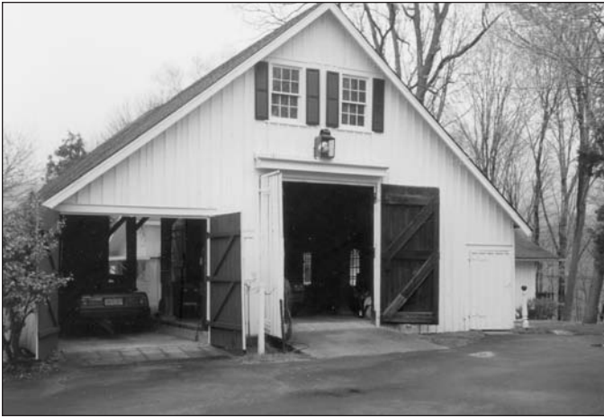
Photo 3. The extant c.1790 classic three bay Bartholf Dutch barn in Mahwah, New Jersey. This barn features nine foot high side walls. It measures 36 feet at its gable wall and 30 feet along its side walls. Exterior siding and gable doors are not original.
