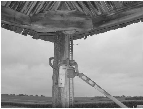
Photo 2. Corner detail showing roof jig in place.
