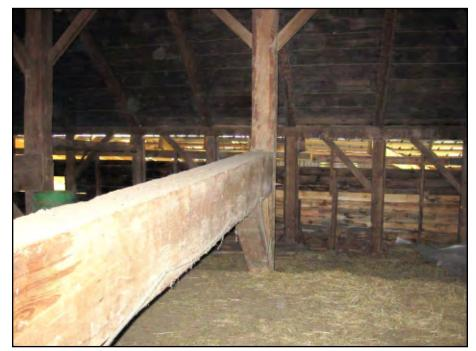
Photo 4. View showing the wall braces.
