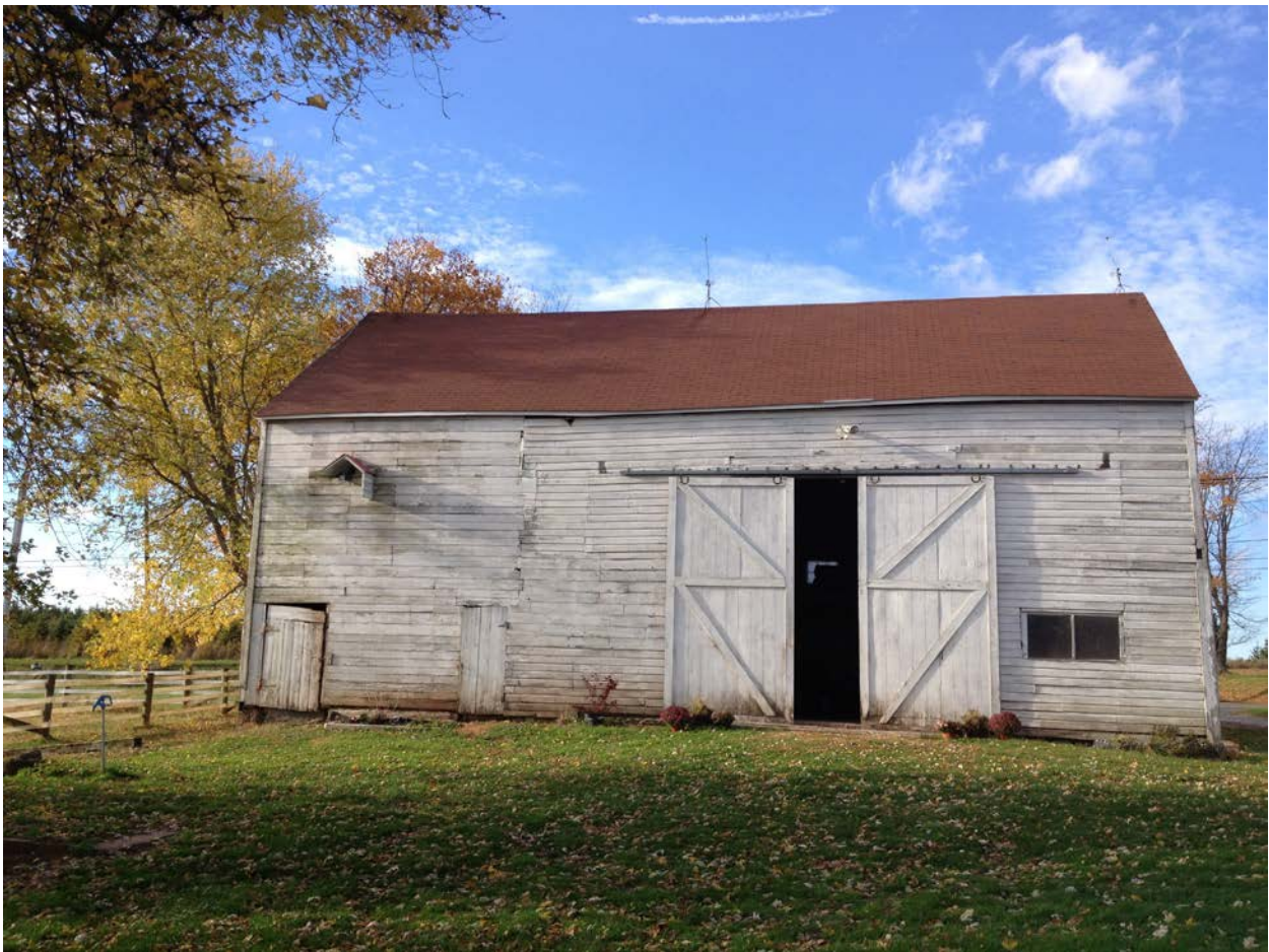
(Photo of the Richard Cain Barn courtesy of Larry LaFevre.)
