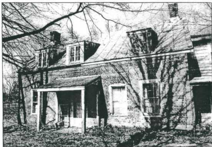
J. Skinkle House, timber frame with brick veneer Route 9-H Kinderhook, Columbia County, NY
