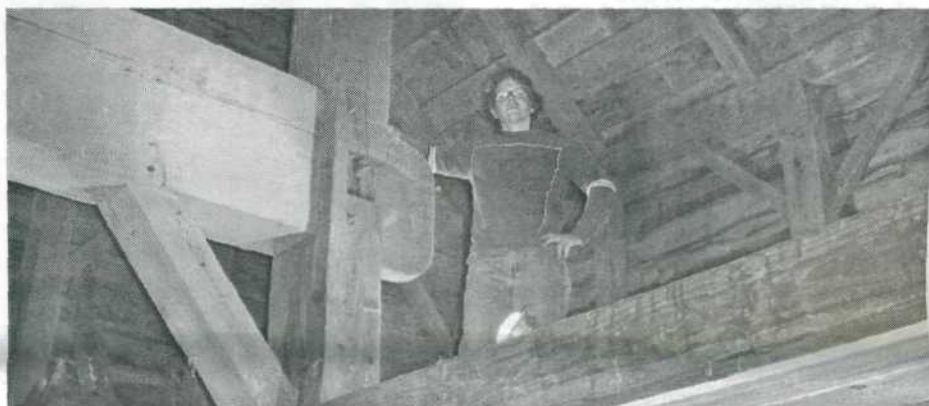
The sheepdog inspects the "huge tongue" on the one of the great anchor beams in a circa 1799 Dutch barn relocated to Anramdale, NY from Fort Plains, NY.
