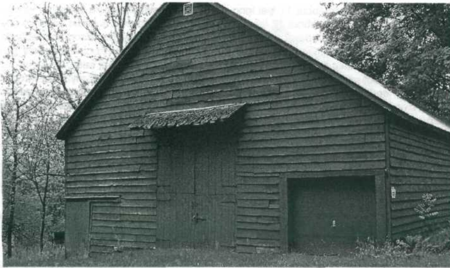
Circa 1820 Brink-Muller variant U-Barn is about one mile south of the Henry Synder barn in the Mount Marion area of Ulster County. This barn is of four-bay construction where the last bay is decidedly longer than the other three individual bays in the barn. This is a view of the far end wall with non-original wagon doors that were likely installed near the end of the nineteenth century.
