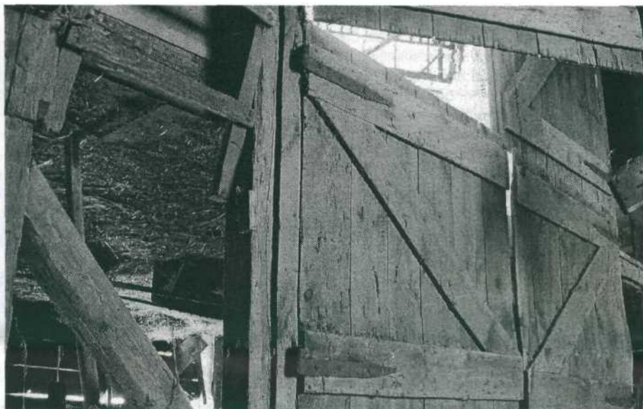
Circa 1825 Henry Snyder variant U-Barn is in the Mount Marion area of northern Ulster County. Above: View of rare original double side by side threshing floor like doors of the last inner bent. Doors swing into the middle bay of barn. Below: View in the far bay that was open to the exterior that apparently allowed hay wagons to back up to the doors that are in line with the last inner bay. At the left edge of the original door is the original mittlemanse or middle-man post that brought the right and left door halves together and held in place.
