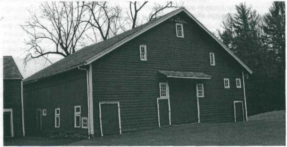
Elmendorph Barn - This variant U-barn that may be circa 1850 near High Falls in Ulster County is the widest of any known extant three-aisle barn in the entire Dutch barn realm. The exterior weather-boarding at the facing gable wall is likely original. The cavernous interior has a unique structure.
