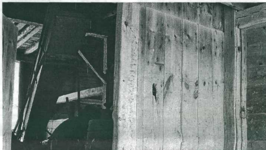
Circa 1825 Henry Snyder variant U-Barn is in the Mount Marion area of northern Ulster County. Above: View of rare original double side by side threshing floor like doors of the last inner bent. Doors swing into the middle bay of barn. Below: View in the far bay that was open to the exterior that apparently allowed hay wagons to back up to the doors that are in line with the last inner bay. At the left edge of the original door is the original mittlemanse or middle-man post that brought the right and left door halves together and held in place.
