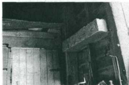
Circa 1820 Brink-Muller variant U-Barn. View of the cut off far end wall lower tie beam that then permitted full wagon drive through status in the late nineteenth century. The cut off tie meets the left post of the wagon doors at the right.
