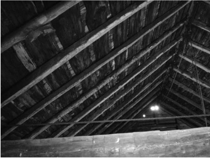
A common rafter system is seen in the Sickler Road barn. Many barn rafters are hewn and are of yellow birch. Above rafters are original roofers with natural waney bark edges. At bottom is upper tie beam of bent.
