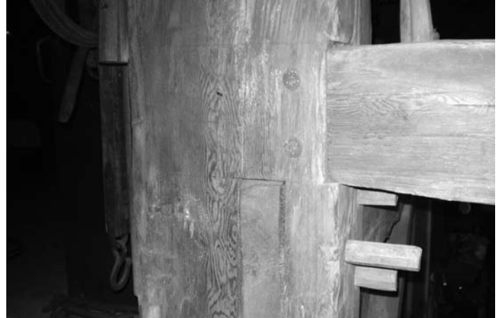
Post of inner bent is seen with outer end or housed tenon of middle tie of bent whose outer edges are chamfered. End of tie is flush with the outer face of post. Post and tie joined with three pegs. At right is longitudinal tie that joins to post with two pegs.
