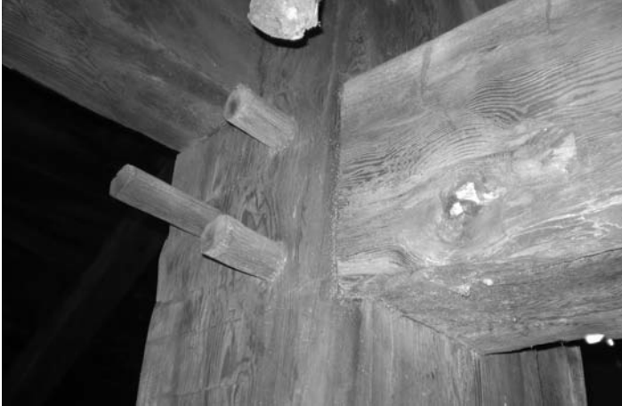
Tie at right unites to post of bent with triple pegs. High placed longitudinal tie at upper left corner joins to post. Beyond at the left is side aisle.
