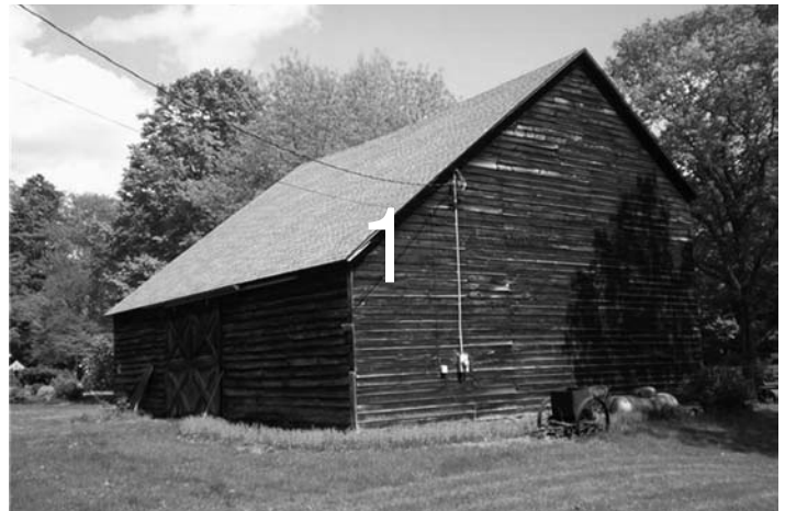
Exterior of Sickler Road two-aisle barn west of Woodstock, Ulster County. Seen is non-original novelty siding on west end wall and regular north side wall siding that is also not original. The north wall includes wagon door of sliding type that is not original.
