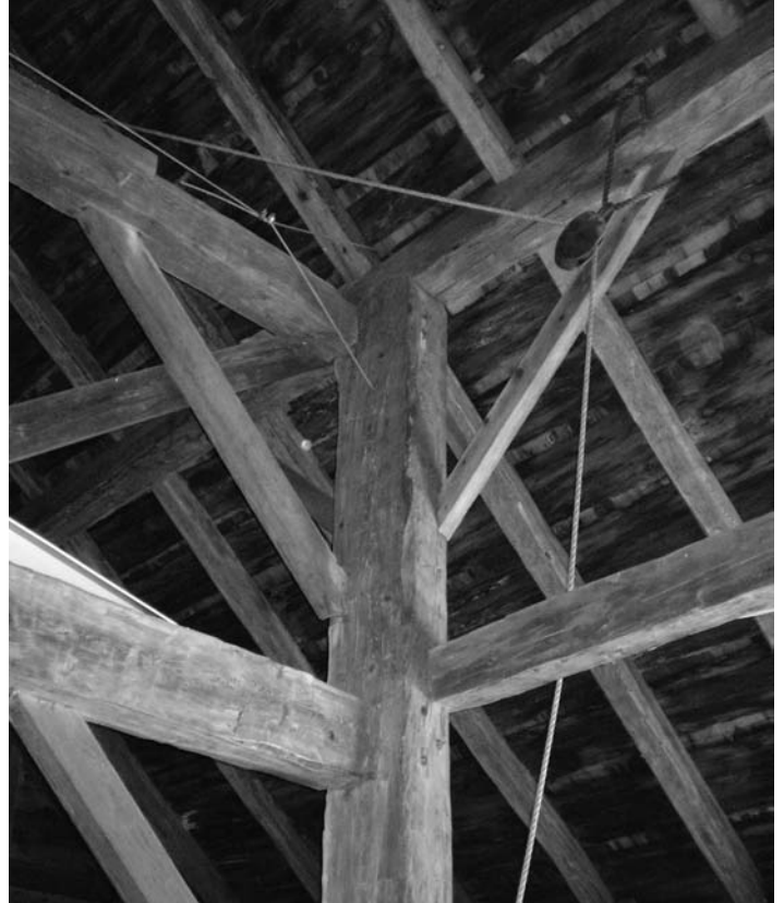
View of many timbers uniting with main post of inner bent at the west side of wagon bay. Purlin plate is seen at top of post with purlin braces seen at either side of post. At left is braced upper tie beam that joins at top of post. Below at left is braced middle tie. At right is longitudinal tie just above level of middle tie that adds stability in barn. Above purlin are common rafters.
