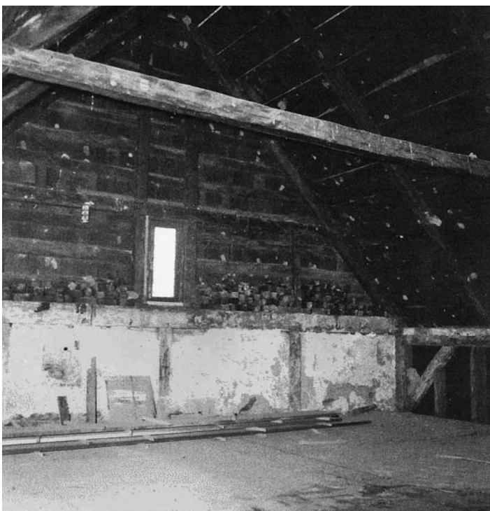
An interior view of the North gable.
