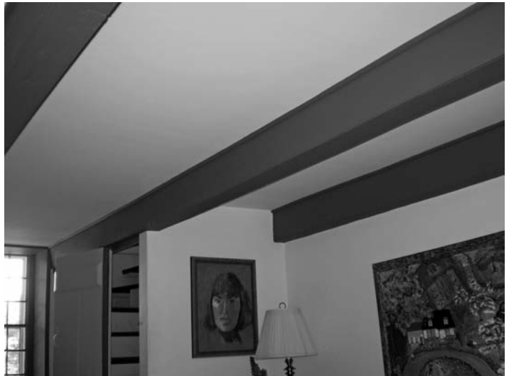
Red joists adorn ceiling of north room on first floor of Conyes house. These joists are quite small by Ulster County standards and are only about 5 by 10 inches in cross section.
