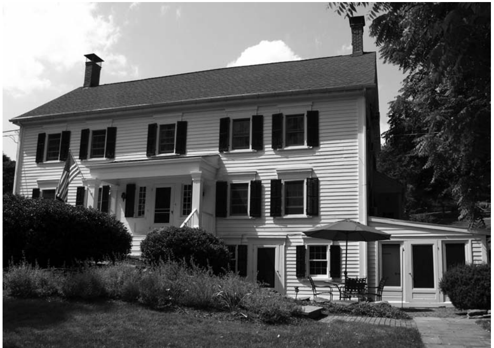
The James Alley House (c.1770) on Todd Hill Road, LaGrange. The exposed cellar on the right side of the house was the kitchen, now converted into a family room.
