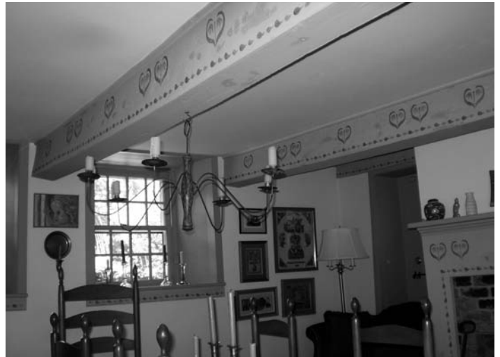
Ceiling joists stretch across full width of house in finished north room in basement. Stenciling was applied to both joists.
