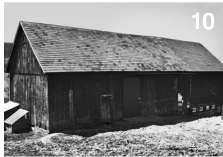
Bellow: English barn at O'Donnell Hill farm. Bottom: Interior detail showing flared posts.
