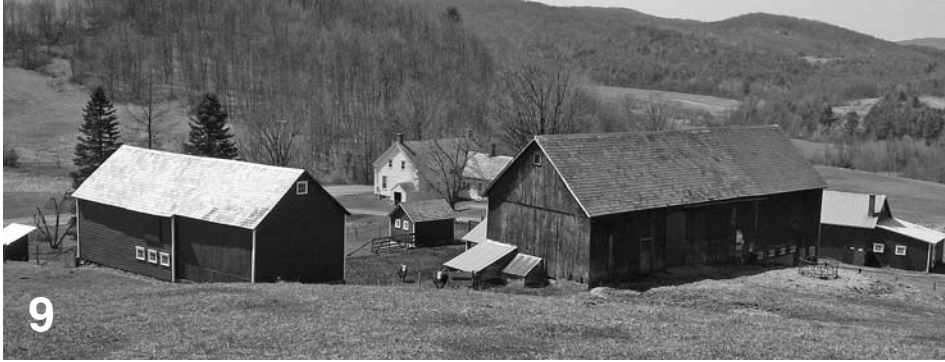
General view of the barns at the O'Donnell Hill farm
