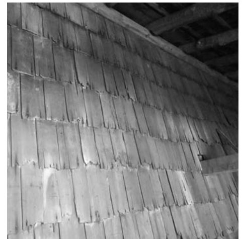
Photo 2: The one exterior side wall of the barn retains much of its original wood shakes. The use of these shakes is a broad regionalism in central New Jersey.
