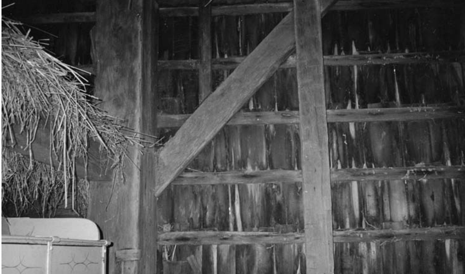
Photo 3: This is an interior view of the one end wall with exterior wood shakes that are secured to thin wood lath. The lath in turn is secured to vertical wall posts or studs.
