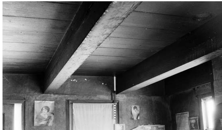
Photo 3: One of the parlors, showing beams (HABS photo).
