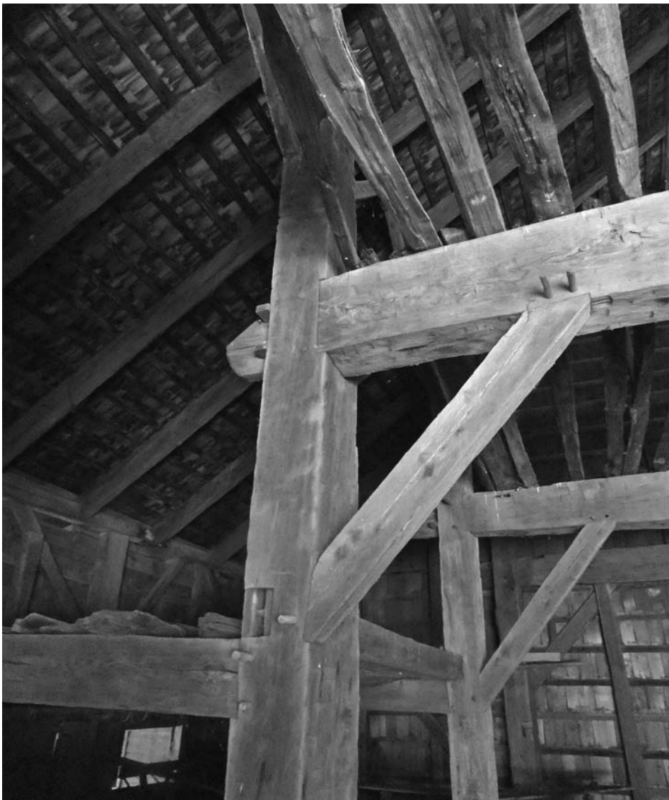
Photo 4: Here are two H-frames with anchor-beam to posts connections. Anchor-beam tenons are double wedged. H-frame braces are medium sized at best.
