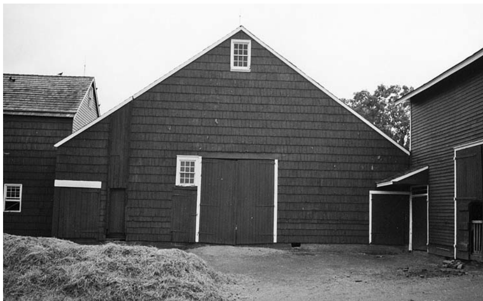
Photo 1: Exterior of the Longstreet Farm three-aisle barn has medium height side walls and a normal height roof peak. Wagon door of two halves is centered on end wall.
