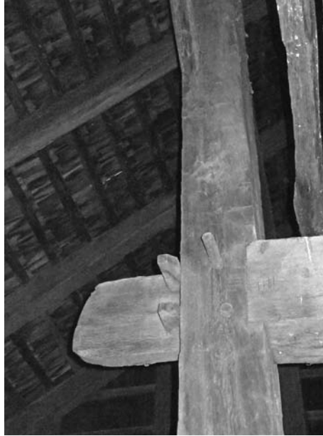
Photo 5: Close up of an anchor-beam to H-frame post connection with the double pegged condition. The timber joint is square shouldered. Anchor-beam tenon contour is basically square. Photo 6: Bottom of an H-frame post is seen with distinctive and prominent notch. Such notches that housed planks for animal mangers constitute a central New Jersey regionalism.
