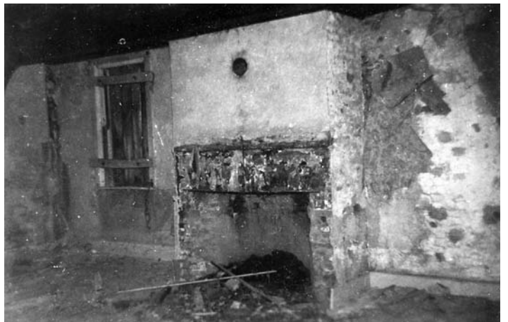
Photo 6: Interior, looking southeast, showing now-removed fireplace, 1956.
