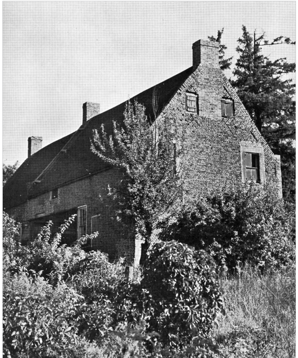
Shown here is a wonderful photograph of the Van Allen House in Kinderhook, Columbia County, New York, taken circa 1940, Prior to the any modern restoration efforts.
