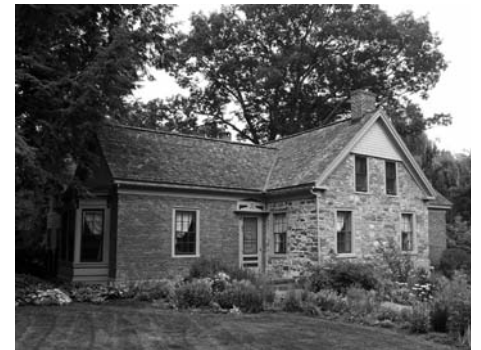
Right across the street at 31 William Street is what appears to be an 18th century stone house with brick additions to the front and back creating an unusual cross shaped footprint.
