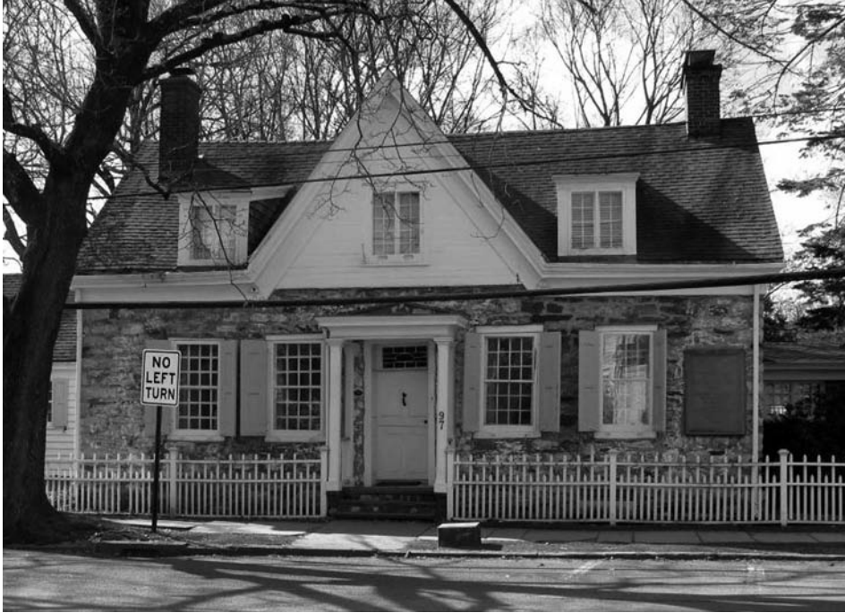
Fig.1 – View of Tobias van Steenburgh House from east. Photo by Jill Fisher, 2012.
