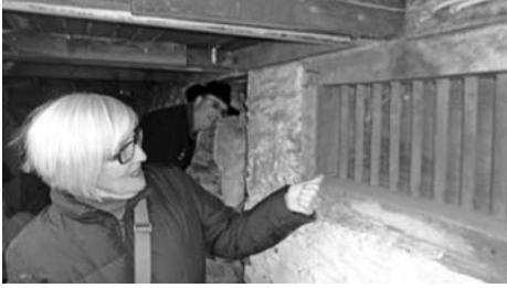
Trustees Maggie MacDowell and Ken Walton in the basement of the Elting House in New Paltz.
