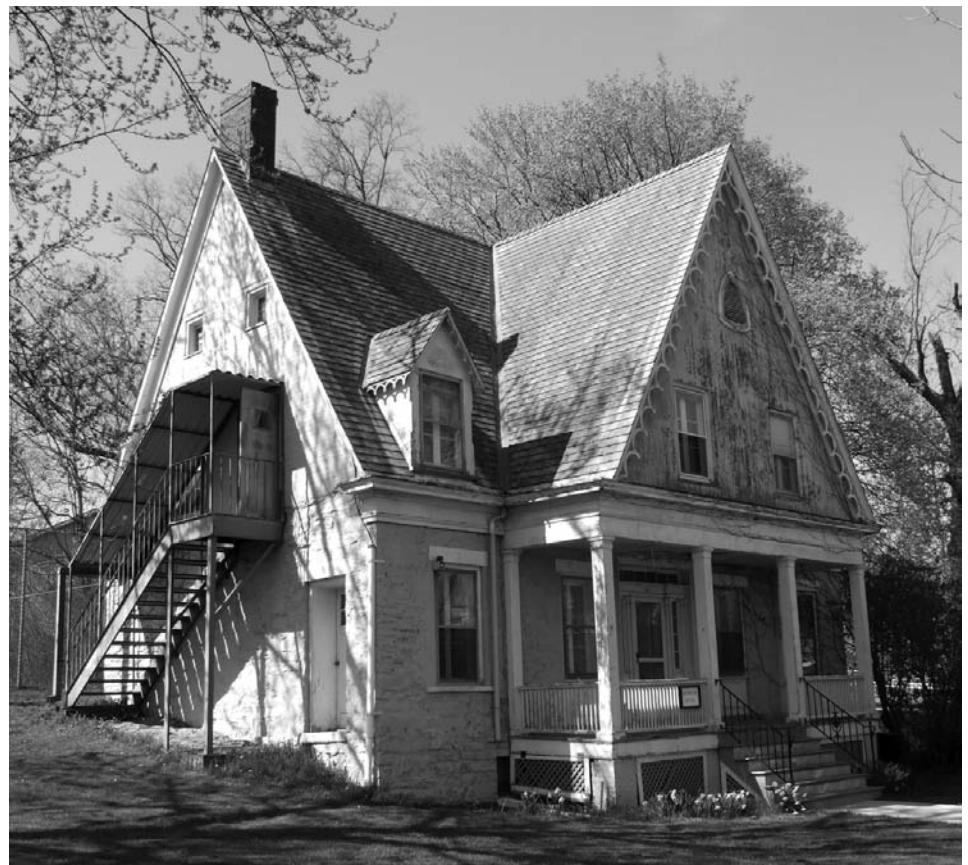
Fig. 2 – Benjamin DuBois House, c. 1740 with extensive later alterations.
