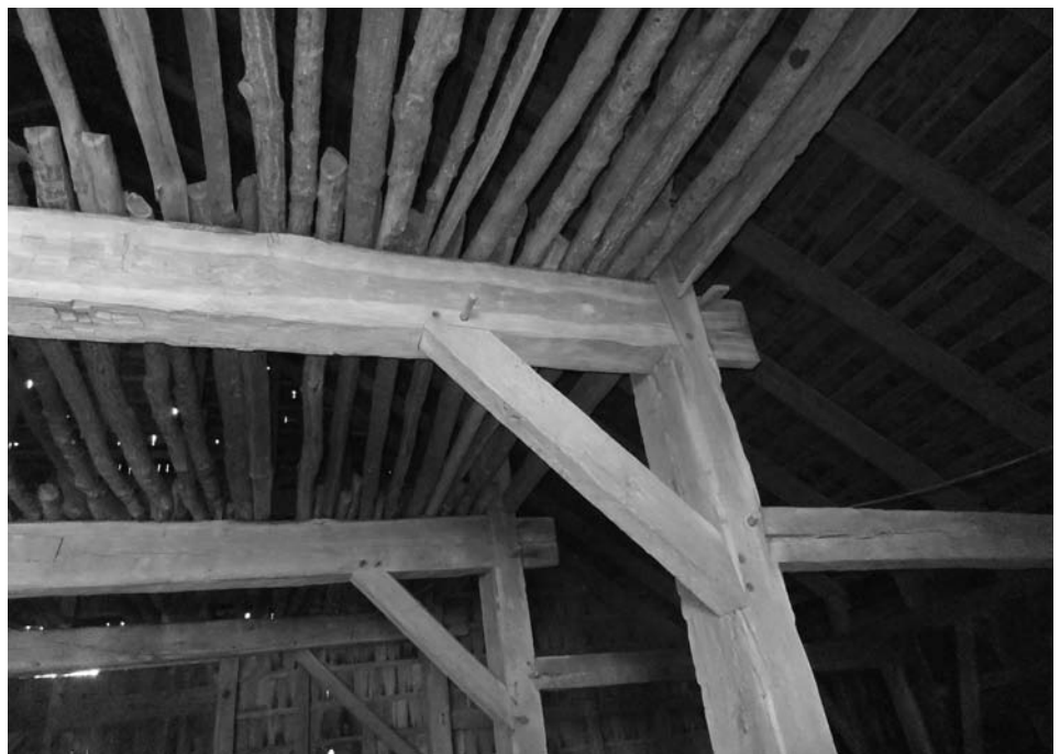
Fig. 3 – Three H-frames are shown at their northwest ends. Note extended tenons of anchor-beams with square contours that are often seen in oak construction. Photo by author.
