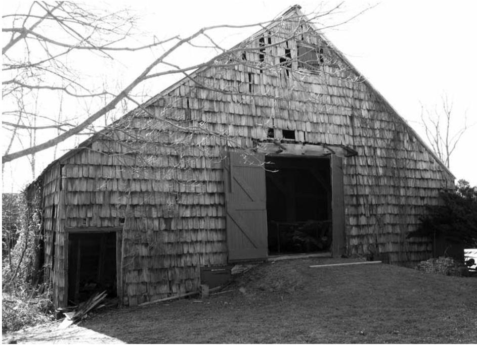
Fig. 1 – View of Schenck Dutch barn from east showing ramp entry and old shingle siding. Photo by Gail Hunton, Monmouth County Parks Department, 2012.
