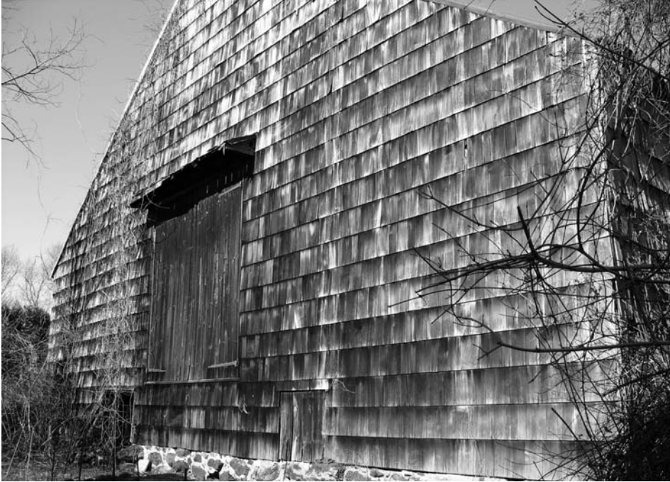
Fig. 2 – View of rear gable end from southwest showing elevated door to threshing floor and doorway into basement to the left of it partially hidden by vines. Photo by Gail Hunton, Monmouth County Parks Department, 2012.
