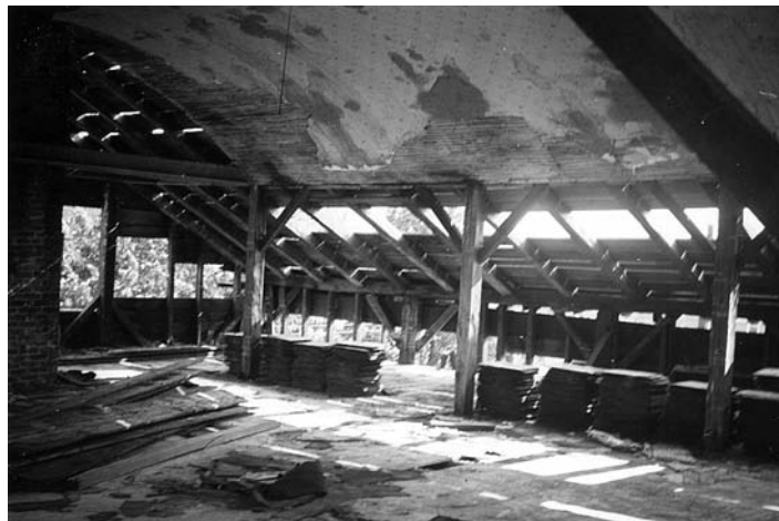
Fig. 6 – View of attic from southwest. The remains of the curved ceiling can be seen, the ends of which rest on the purlins.
