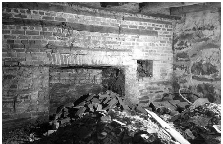
Fig. 2 – Basement kitchen fireplace, looking northwest. Note the parallel hewn logs of small size supporting the first floor. The room had been stripped of its fittings and finishes by this time.
