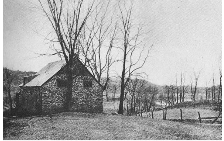
Fig.8: Johannis J. Van Wagenen House, 1775, not extant. Photo from Helen Wilkinson Reynolds, Dutch Houses in the Hudson Valley Before 1776 (1929), 38.
