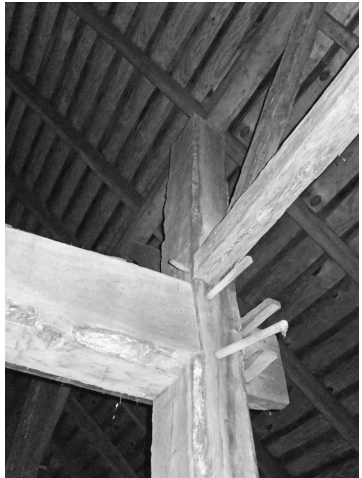
Fig. 2 – View of anchor beam to H-frame post union of inner bent. Union is double pegged and double wedged. View includes five foot long upper H-frame post extension or verdiepingh . Such short post extensions are typical of a number of pre-Revolutionary-War-era barns, especially in southern New York and New Jersey. All timbers are of oak that is typical of most barns in New Jersey.
