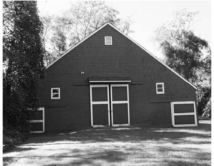
Fig. 1 – View of Couvenhoven Dutch barn looking west showing its very broad end wall indicating a pre-Revolutionary-War-era of construction.
