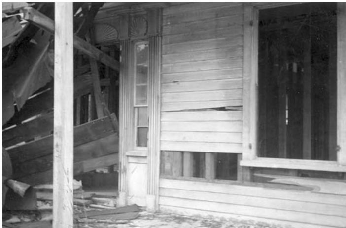
Fig. 3 – Detail showing the front door and a sidelight, looking west-south-west. The applied shell-form decoration was a feature of the lintels on both the east and south (that is, street) elevations. It is not known if they were also used on the secondary facades.
