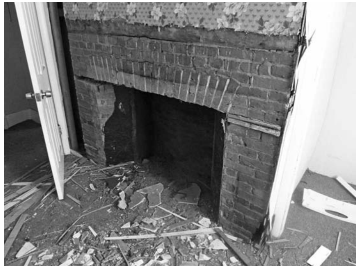
Fig. 10 – View of fireplace in front room on first story, 2012. Photo by J-F De Laperouse.
