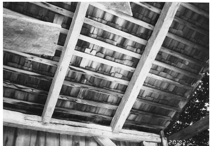
Fig. 3 – View of underside of roof showing rafters, wood shingles and oak lath. Note bottom ends of rafters are fish-mouthed onto wall plates. Photo by Greg Huber, 1992.
