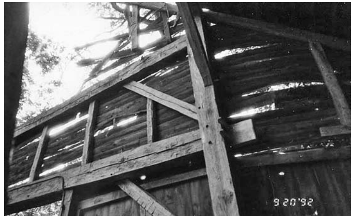
Fig. 7 – View of house-side end wall showing anchor-beam with square through-tenon and anchor beam brace at its right end. Above anchor beam is an upper tie beam and brace positioned near the top of the post. Photo by Greg Huber, 1992.
