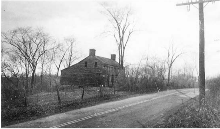
Fig. 1 – View of House #1 believed to be looking north-northwest (all photos and drawings by Carl Erickson, 1956 unless otherwise indicated).
