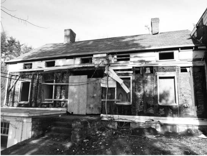
Fig. 7 – View of front facade from south with siding removed, 2012. Photo by J-F De Laperouse.
