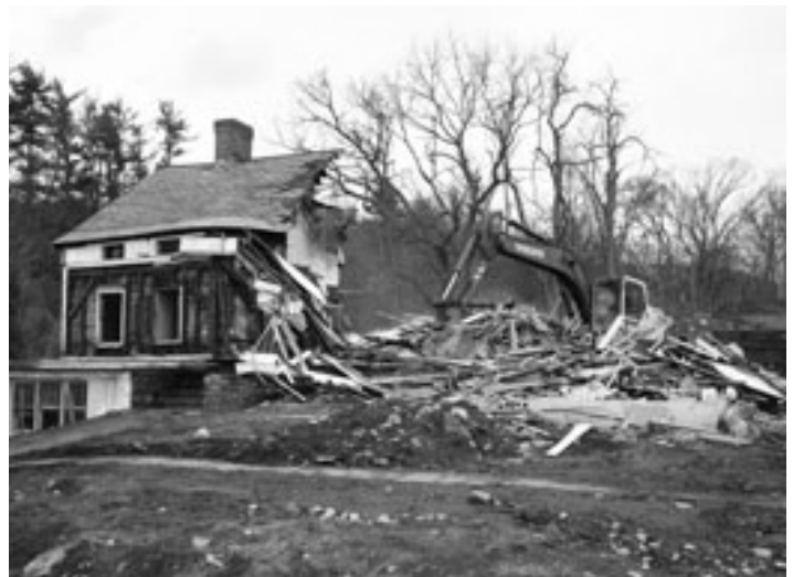
Fig. 11 – View of house being demolished, 2012. Photo by J-F De Laperouse.
