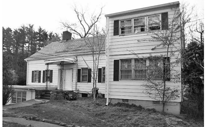
Fig. 1 – View of house from southeast, 2009. Photo by Sullivan Architecture, Thornwood NY.
