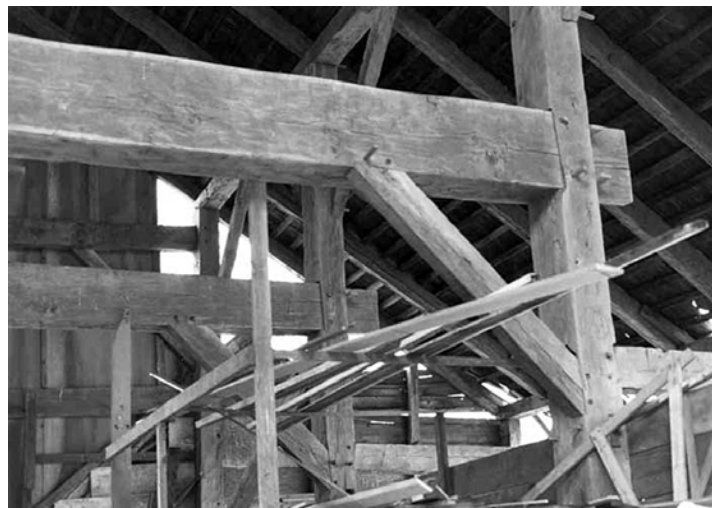
Fig. 5 – View of interior showing joint sections of two H-frames and part of one side aisle. Note distinct square profile of anchor-beam tenon extensions. H-frame braces secured at each end with double pegs. Photo by Gail Hunton, 1981.
