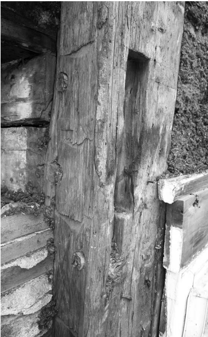
Fig. 8 – Detail of H-bent joint on east side of front façade, 2012. Photo by J-F De Laperouse.
