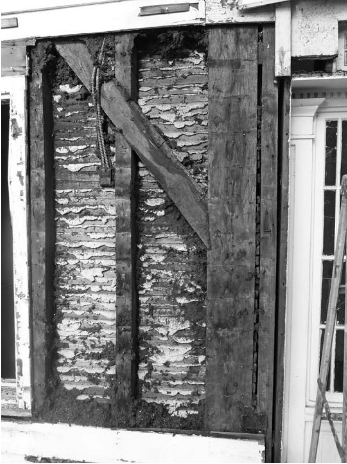
Fig. 9 – Detail of framing on west side of front façade, 2012. Photo by J-F De Laperouse.
