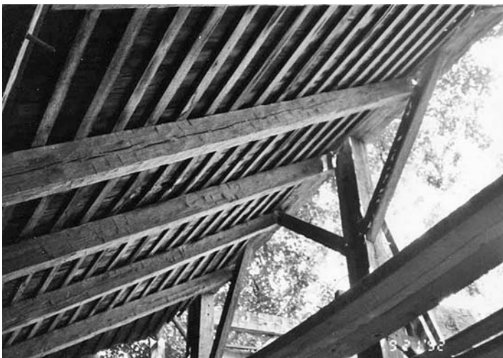
Fig. 2 – View of rafters remaining over one side aisle; sections above the purlin having collapsed onto floor of barn. View includes two H-frame posts with their attendant purlin braces. Photo by Greg Huber, 1992.
