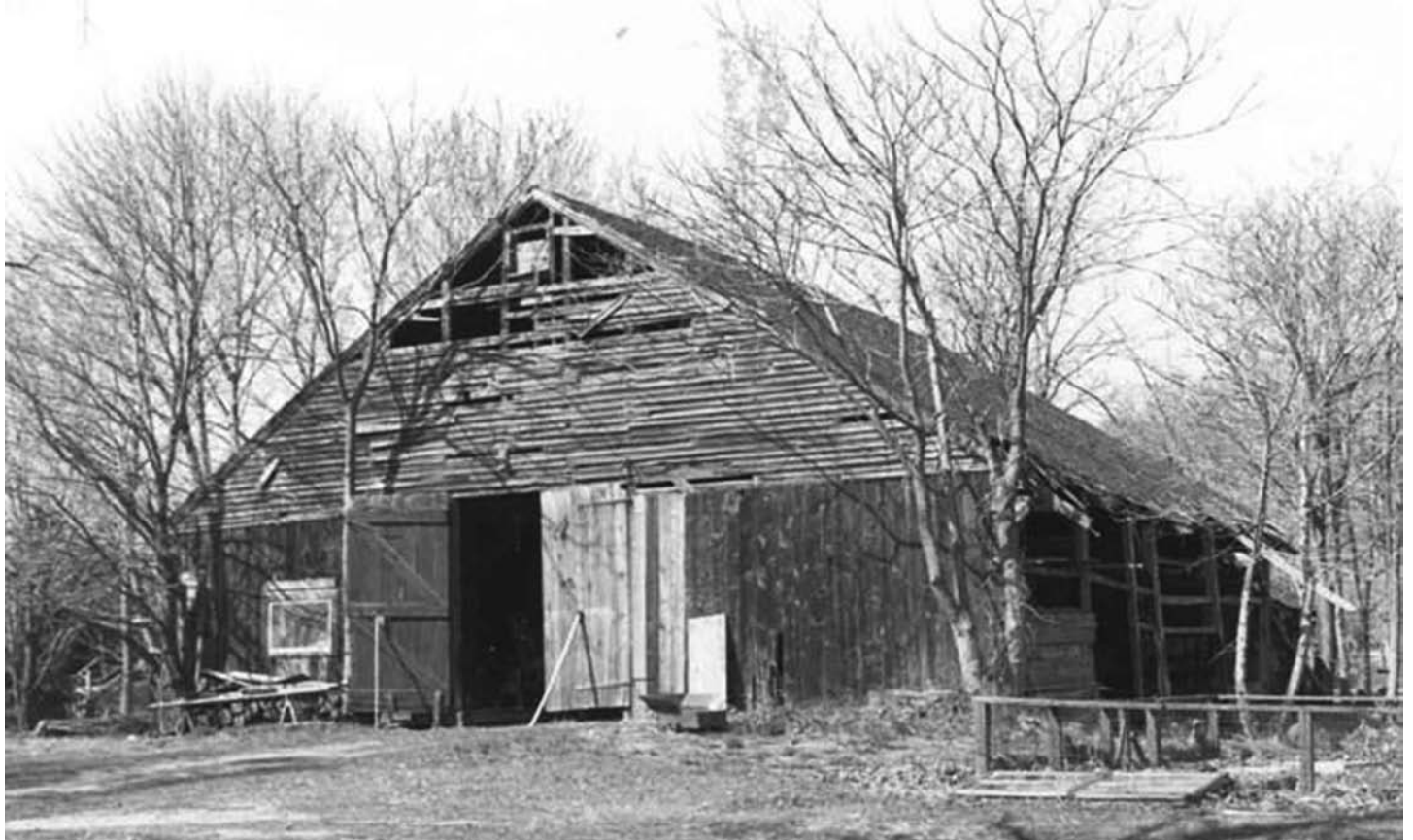
Fig. 1 – The Hendrickson three-aisle barn, Crawford Corners Road, Holmdel NJ, c. 1790. Note deterioration of eave wall on the right. Photo by Gail Hunton, 1981.
