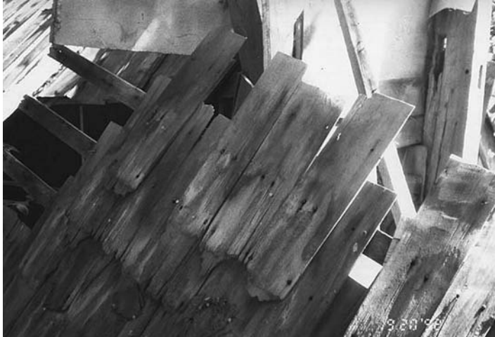
Fig. 4 – View of original roof shingles with sections exposed to weather reduced to nubs. The shingles were secured to roof lath with wrought nails. Section of roof covering shown here had fallen to ground. Photo by Greg Huber, 1992.
