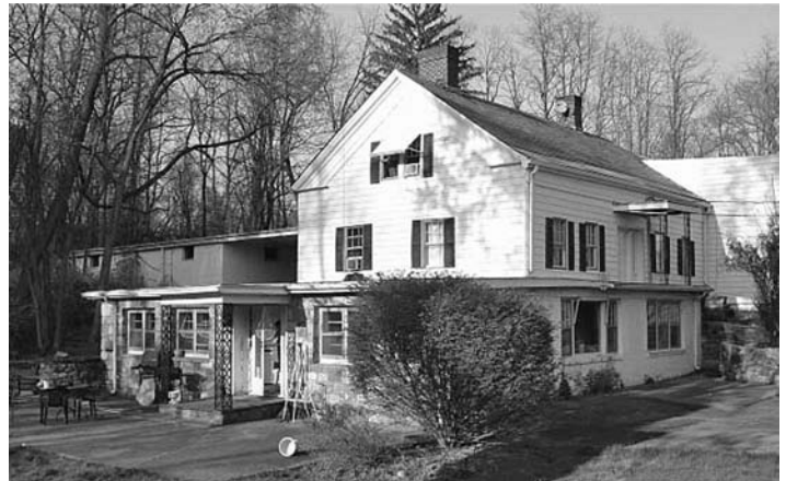
Fig. 5 – View of house from southwest, 2009. Photo by Sullivan Architecture, Thornwood NY.
