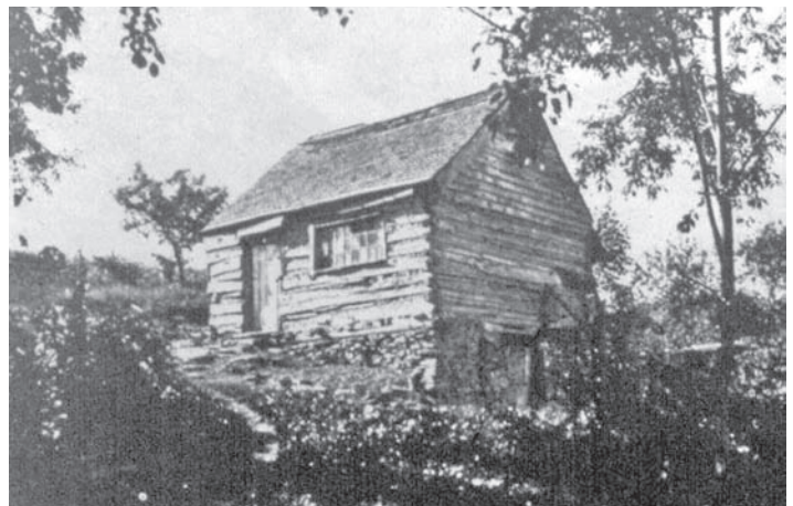
Fig. 11 – Unidentified log house, Town of Hurley, Ulster County, NY. From Picturesque Ulster , 115.
