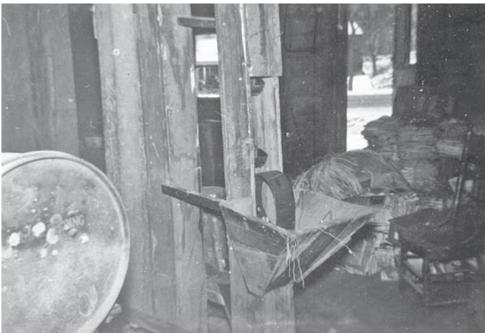
Fig. 5 – Interior view showing equipment, winter 1955/56.
