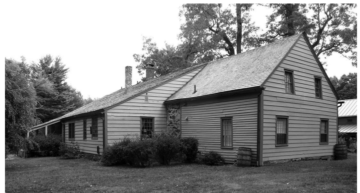
Fig. 3 – View of house from northwest. Photo by Neil Larson, 2014.
