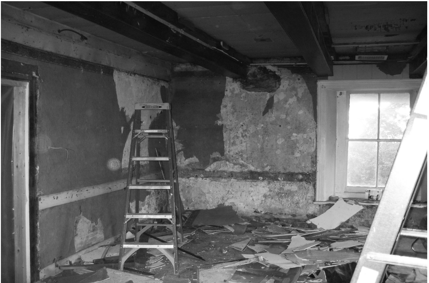
Fig. 5 – Living room during demolition. The beams were painted with many coats of paint. Note the BX wire, top left, coming through then back into the 11" beam.
