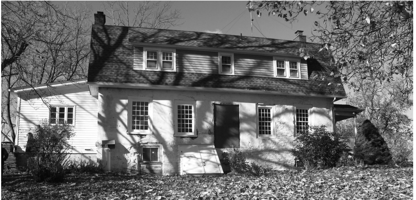
Fig.1 – View of house from east. Photo by Neil Larson, 2014.
