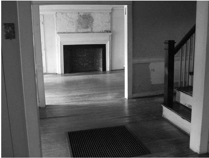
Fig. 1 – View from living room into dining room. Note the 18th c. mantel, juxtaposed with 20th c. heating grate, newel post and archway mouldings.
