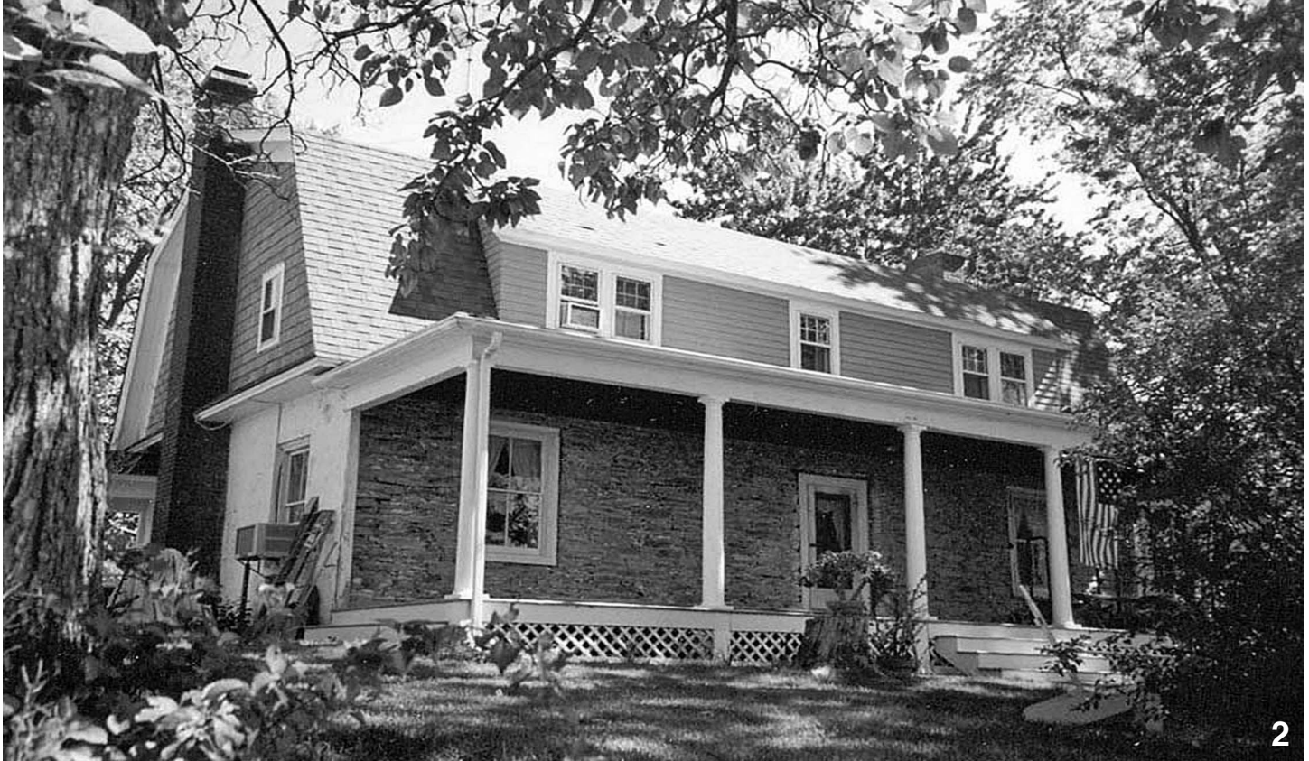
Fig. 2 – View of house from northwest. Photo by Neil Larson, 2001.
