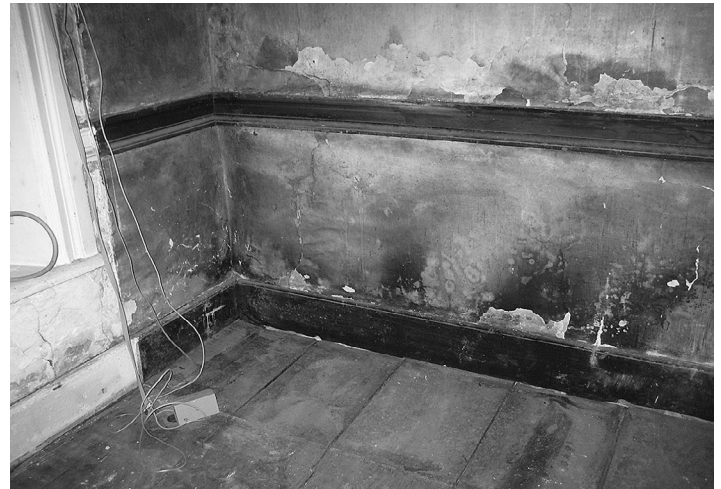
Fig. 3 – Original chair rail, baseboard and plaster exposed beside dining room fireplace.
