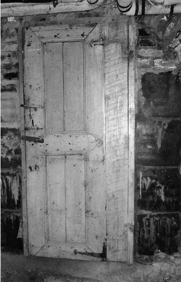
Fig. 1 – View of panel side of door in Grace-Hornbeck House, Accord, New York. Photo by author, 2015
