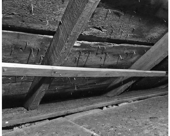
Fig. 6 – Detail of rafter where it joins the purlin.
