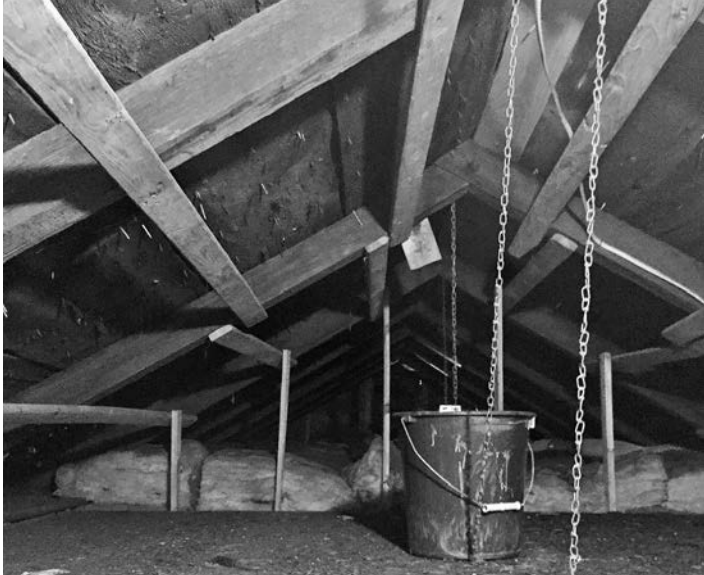
Fig. 5 – View of upper roof frame.
