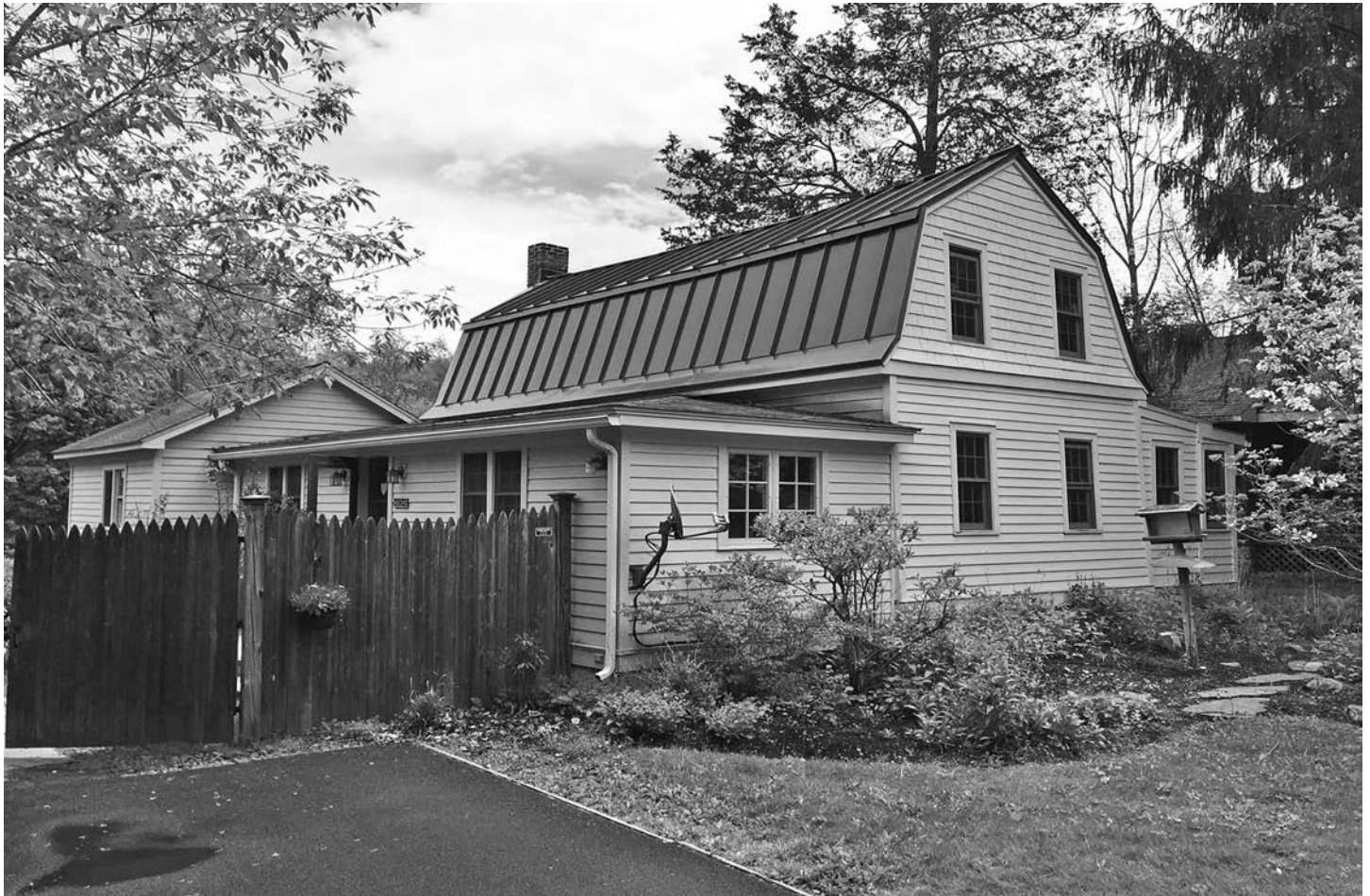
Fig. 1 – View of house from NW. The wing on the right was a porch bumped out and enclosed as a room in the 1990s. The one on the left is a more recent addition.
