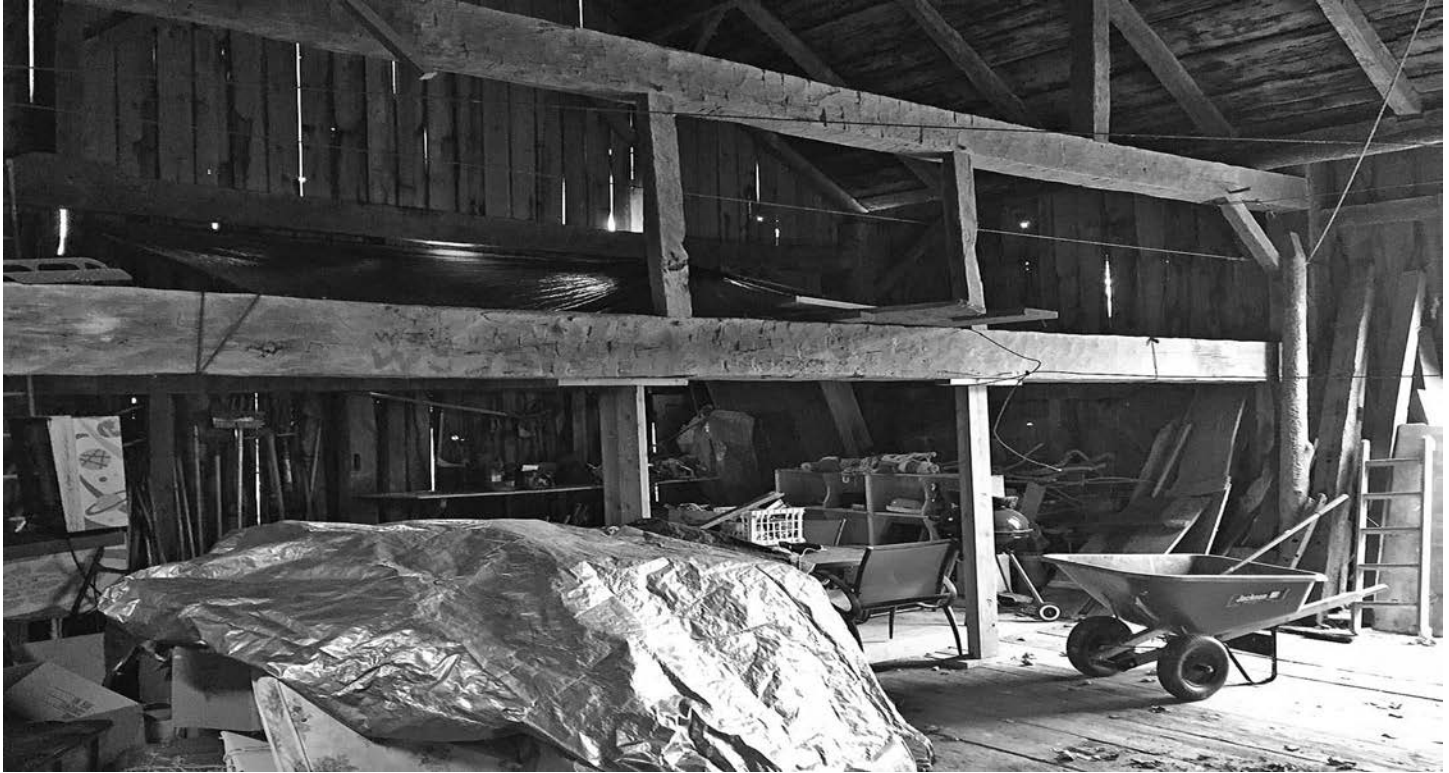
Fig. 7 – View of barn interior and swing beam. Photo by Neil Larson, 2017.
