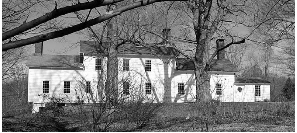
Fig. 1 – Hauver-Sleight House, Schoolhouse Rd., Clinton, ca. 1760 and later. Photo by Neil Larson, 2013.
