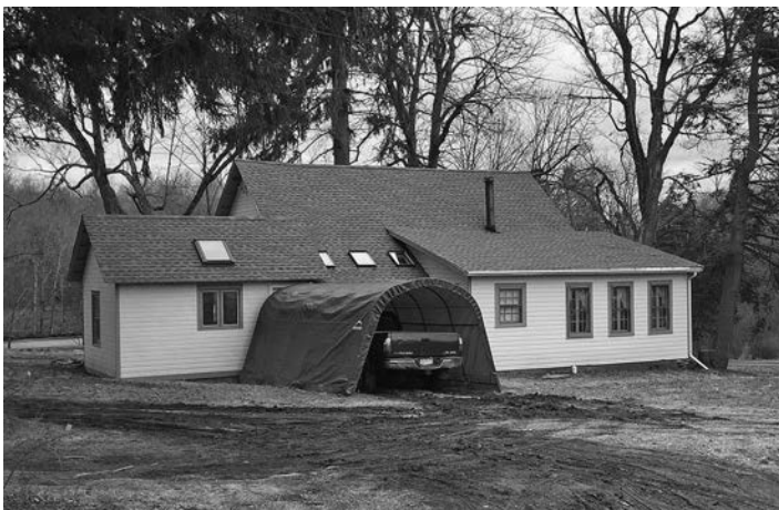
Fig. 10 – View of house from northeast. Photo by Neil Larson, 2017.
