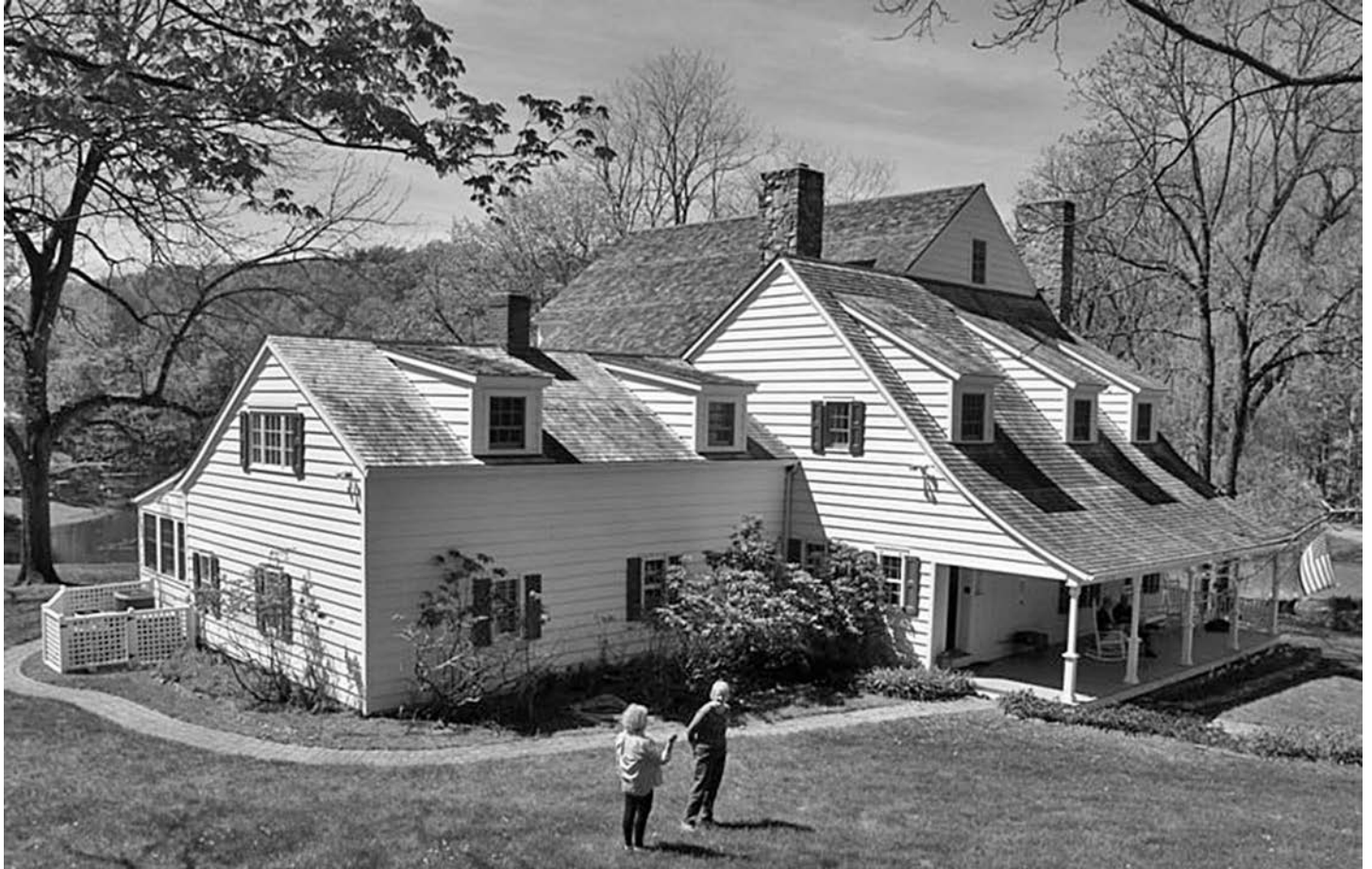
Fig. 2 – Christie-Crapser House, Schoolhouse Rd., Clinton, ca. 1760 and later. Photo by Neil Larson, 2013.
