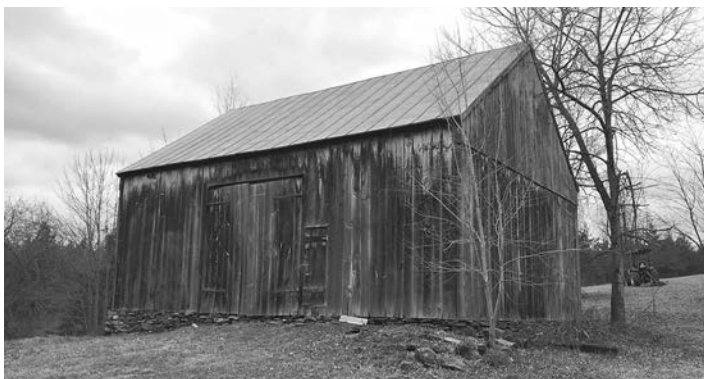
Fig. 6 – View of barn from southeast. Photo by Neil Larson, 2017.
