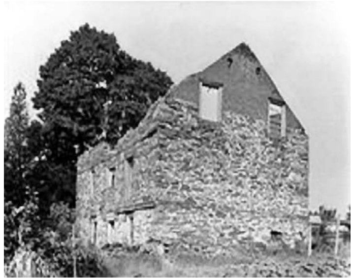
Fig. 3 – Ruins of Johannes & Catherine Rau House, 1766 (not extant). Historic American Building Survey, 1933.
