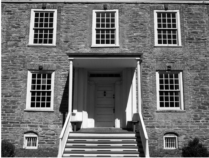
Fig. 7 – Van Cortlandt Mansion, detail of front façade showing brickwork around windows. Photo by Neil Larson, 2005.
