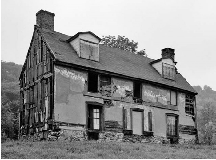
Fig. 9 – John Haskell House, New Windsor, Orange County, NY, ca. 1721. Photo, 1978. This house was demolished in the 1980s. HABS NY, 36-NEWI, 1-.
