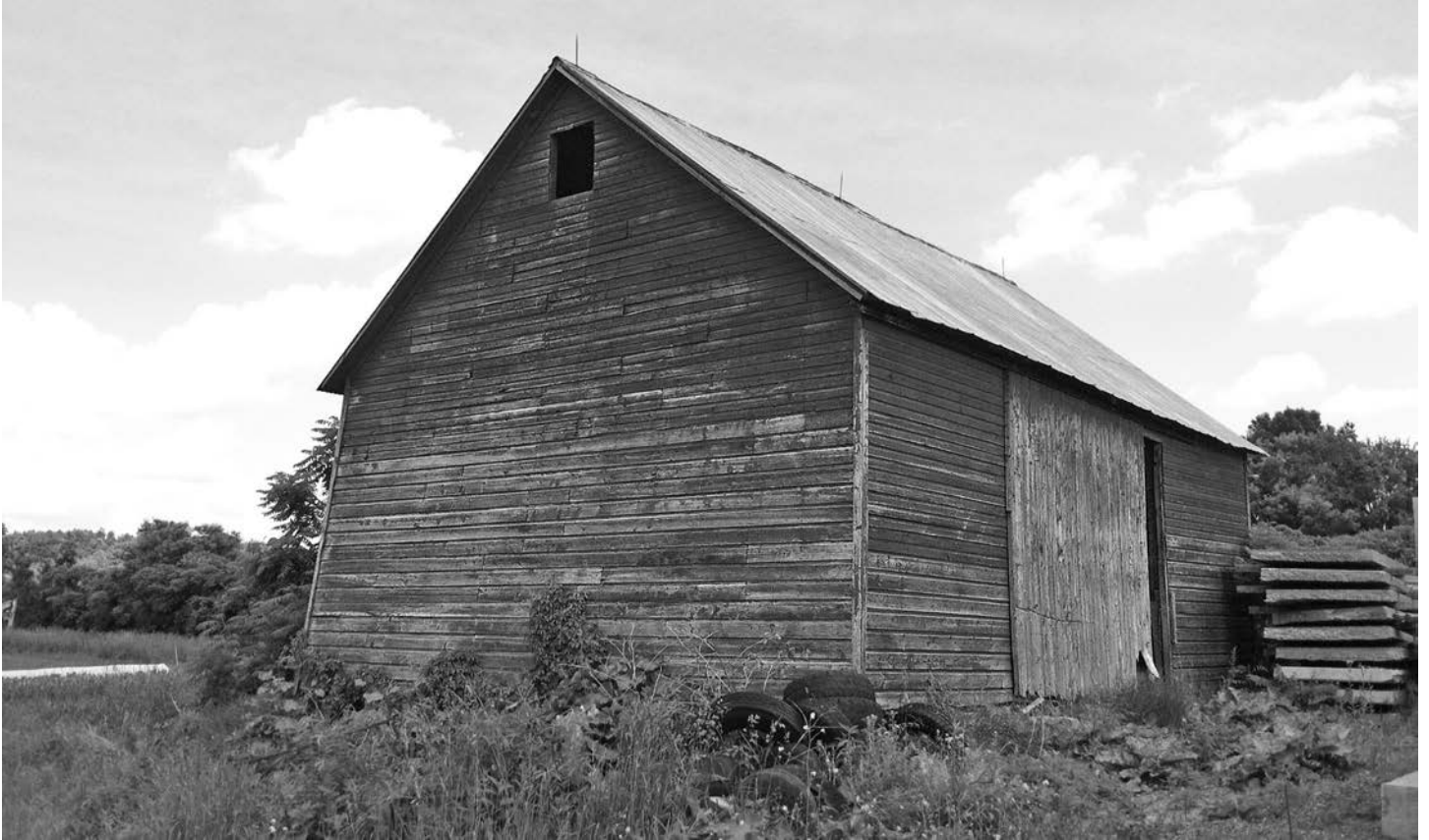
Fig. 4, and Fig. 5 (next page) – Small three-bay barn, Easton. Combines all dropped tie-beam bents with a roof-framing system of New England precedent.
