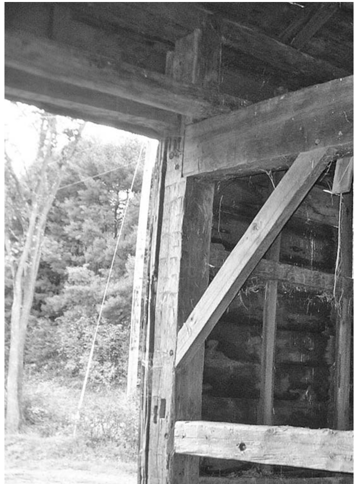
Fig. 8, and Fig. 9 (below) – Barn, Salem vicinity. Example of the standard type employing both English tying joints and dropped ties. (Photos by William Krattinger)
