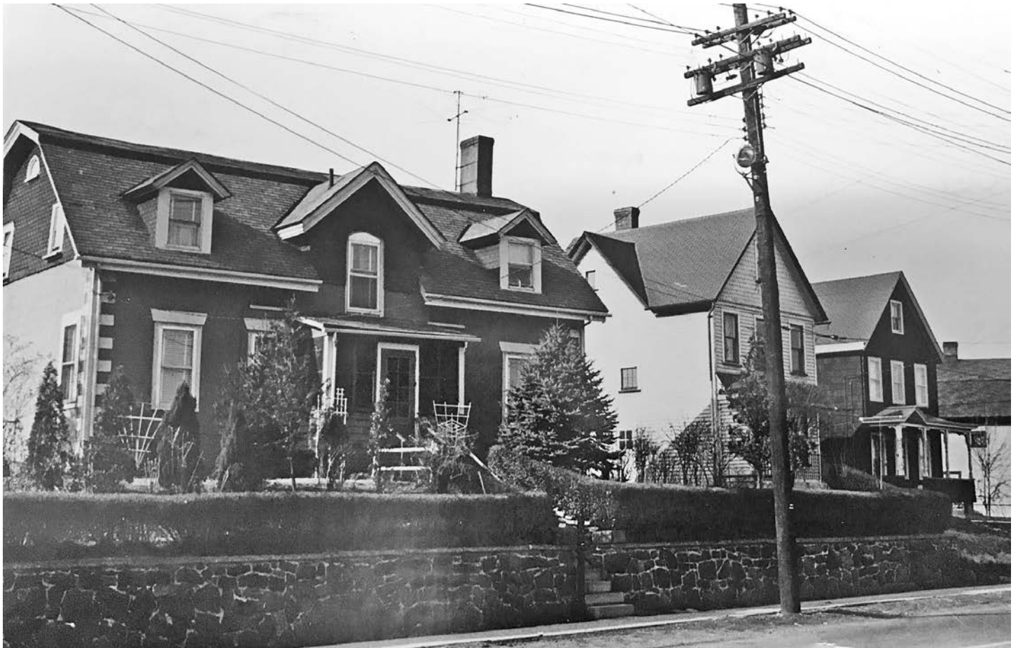
Fig. 5 – Streetscape with house in foreground, ca. 1950. (Author's collection)
