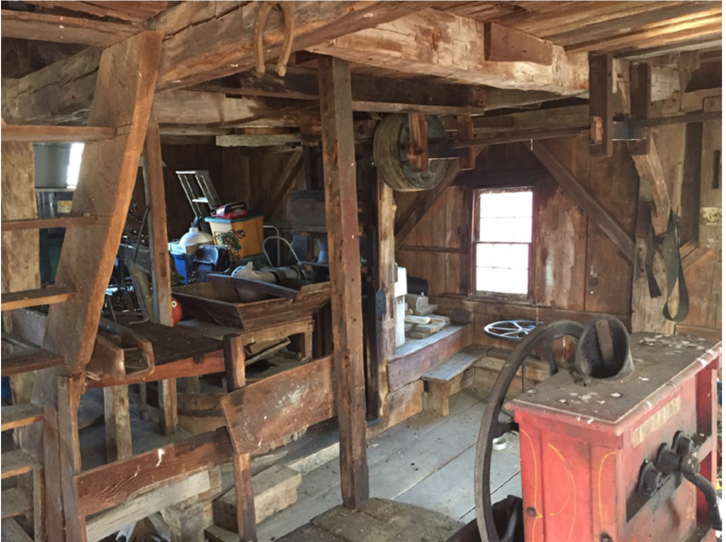
Fig.2: View of interior, second floor. Photo by N. Larson.
