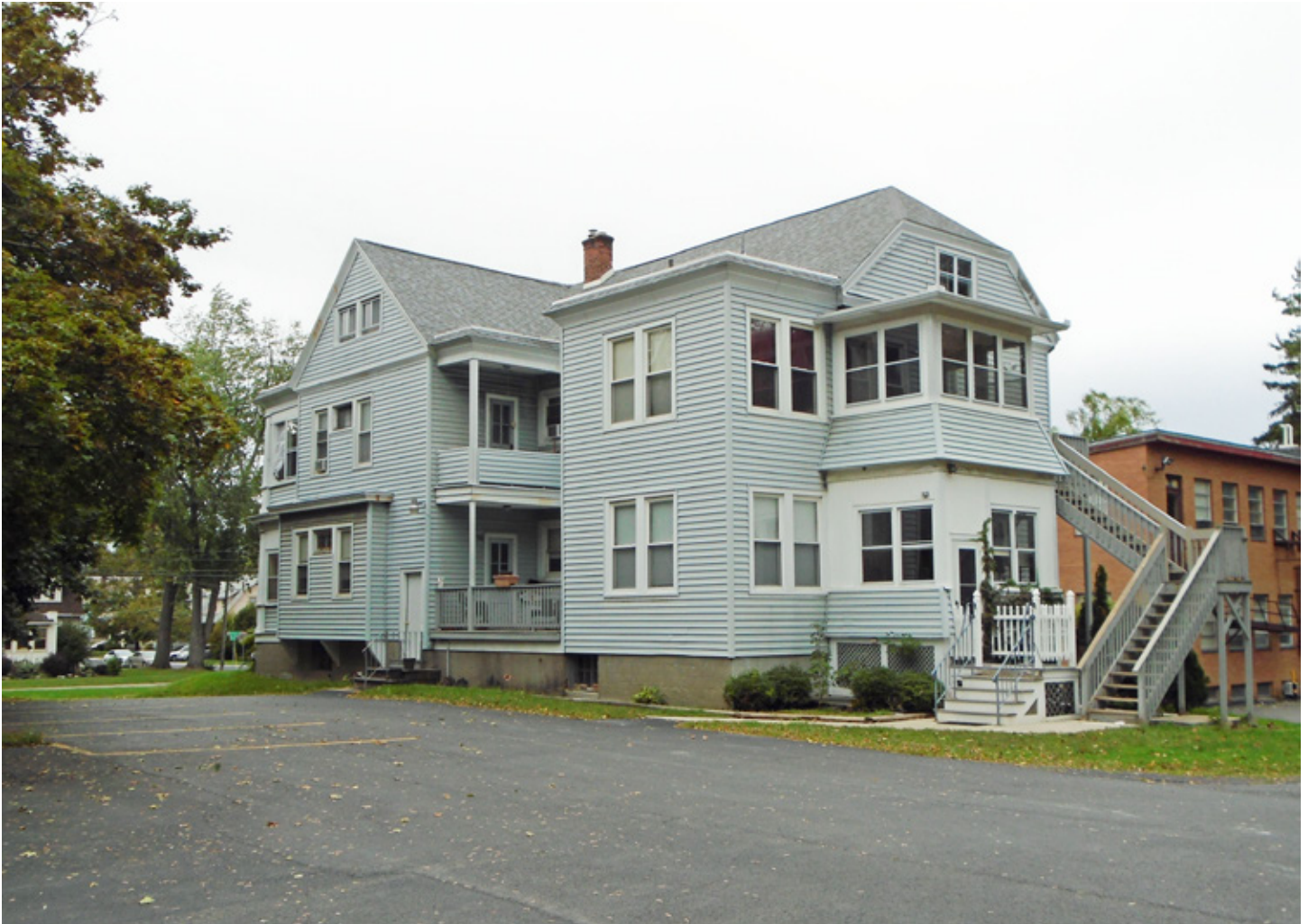
Fig.17. View of the replacement “White Hall” house, looking west (photo by Marcela DiVirgilio, September 2019).
