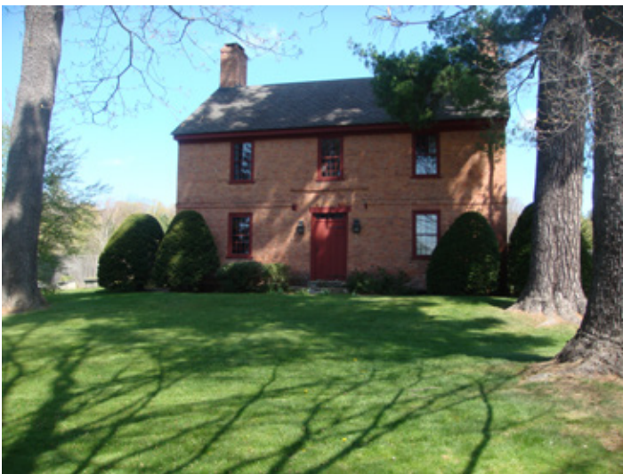
Fig.10. The Jonathan Whiteside house, Cambridge, Washington County, NY, 1791-92 (photo by Bill Krattinger, April 2012).
