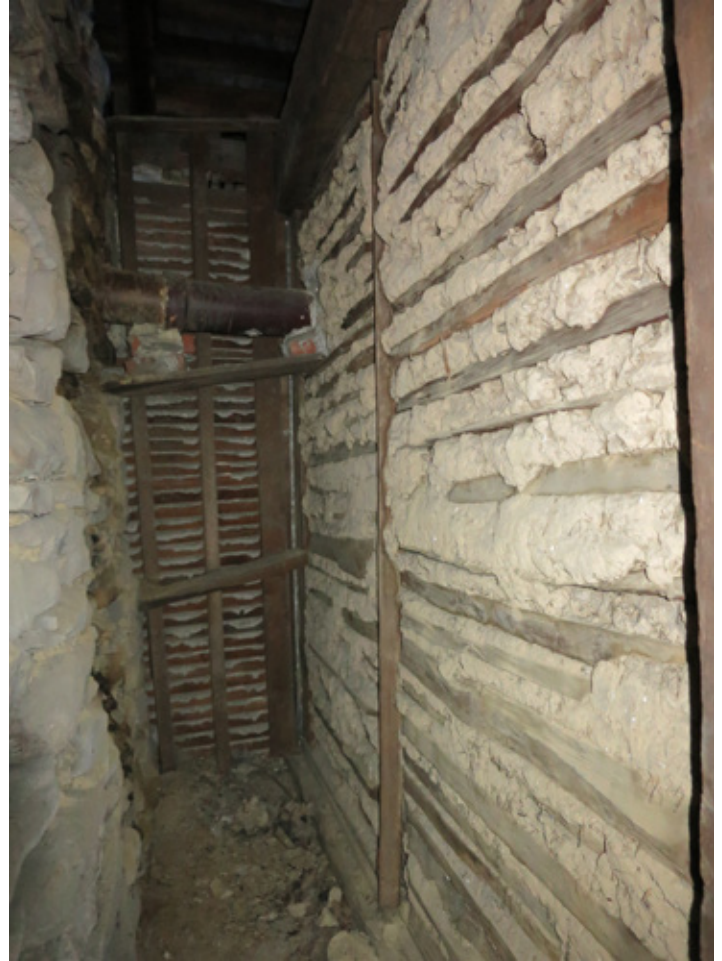
Fig.7: View of mud-packed wall, second floor, from chimney space.
