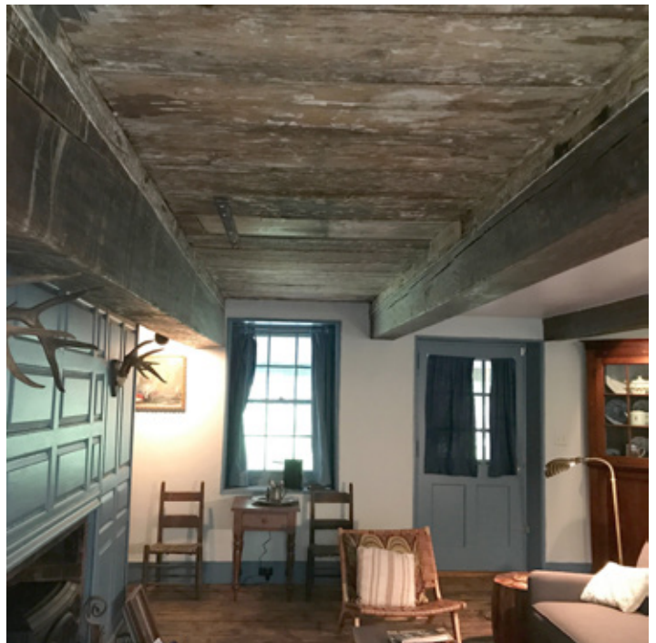
Fig.8: View looking east in south parlor showing massive beam that supported chimney jambless fireplace on left. Photo by Rachel Coates, 2019.
