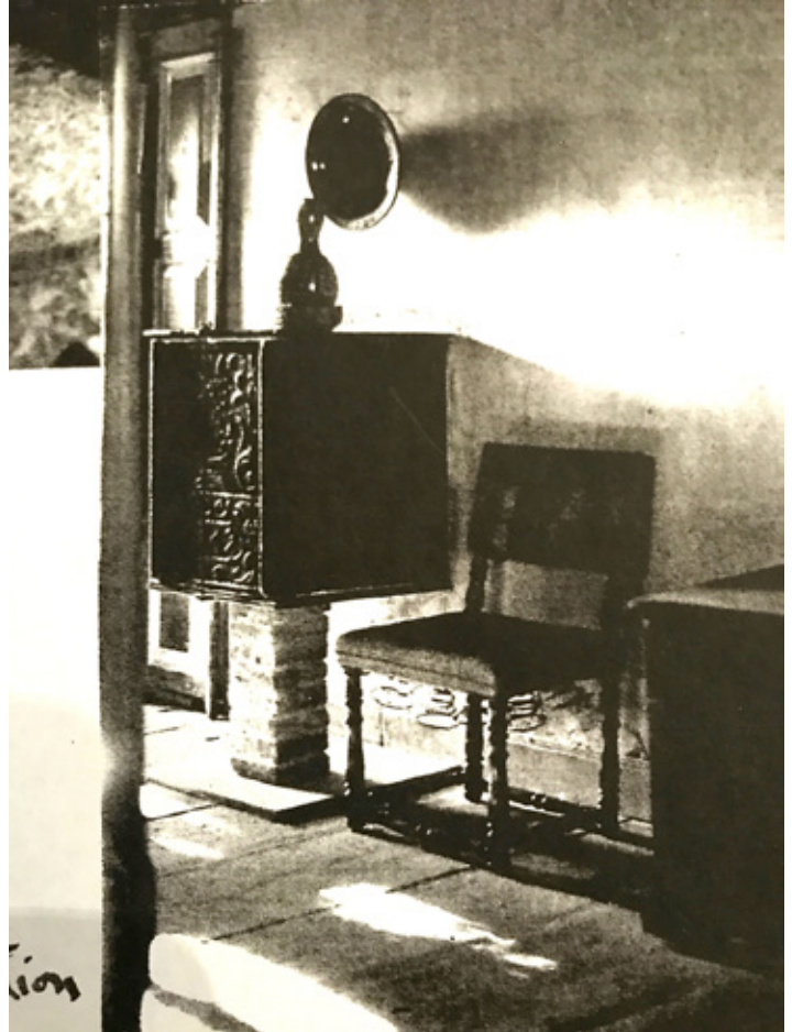
Fig.7: Example of five-plate stove embedded in back of jambless fireplace in adjoining room. Photo courtesy John Stevens.
