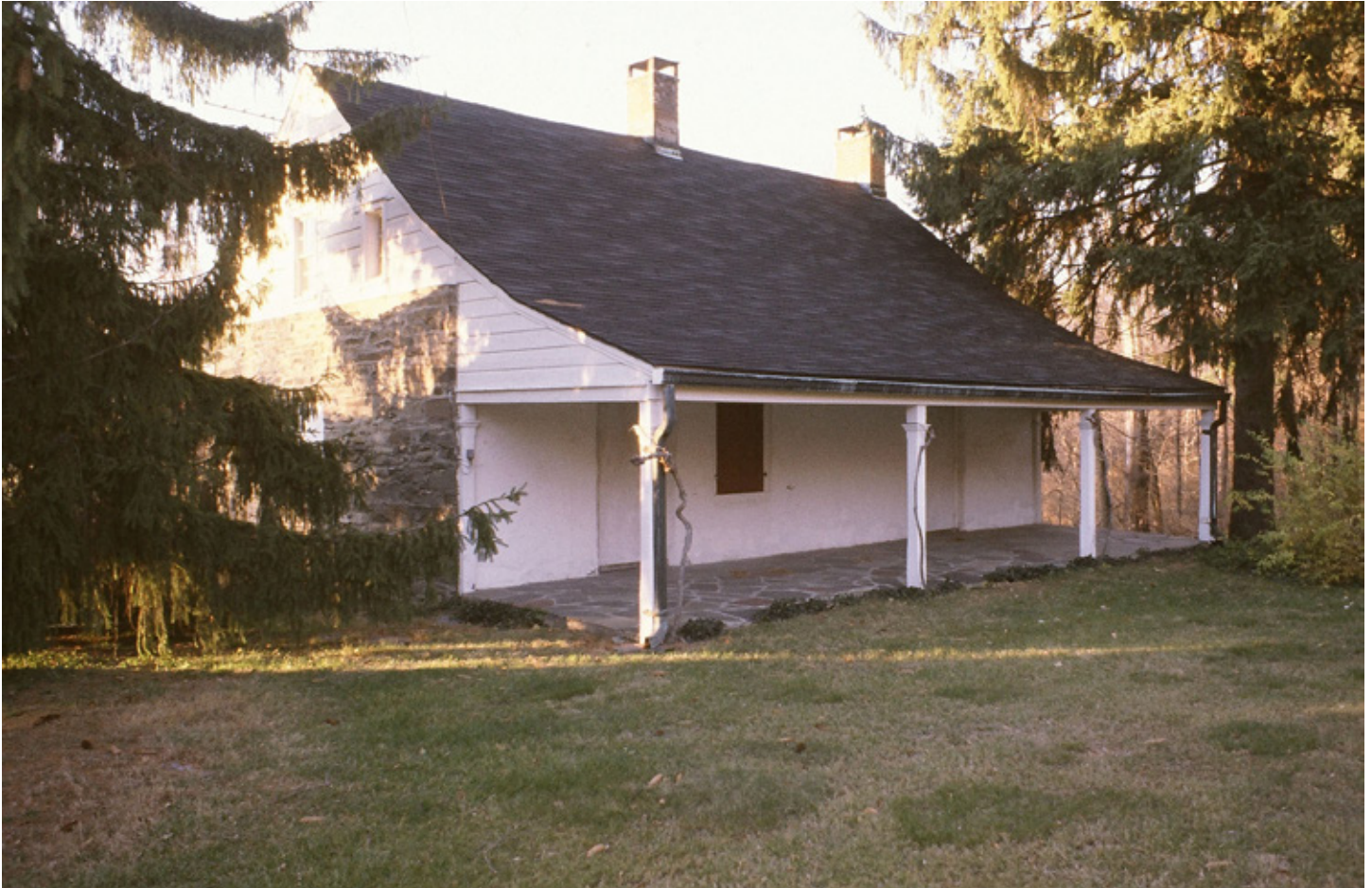
Fig.1: View of house from southeast. Photo by Joe Alper, 1969. Color print used for Landmarks of Dutchess County, 1683-1867; Architecture Worth Saving in New Your State (NY: New York State Council on the Arts, 1969), p.48.
