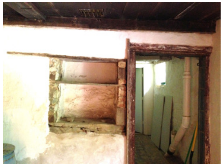
Fig.3. Detail of south wall basement kitchen showing timber-frame doorway and built-in shelves; ceiling beam to support upper-story stove visible in upper left corner of image. Photo by Rachel Coates, 2019.
