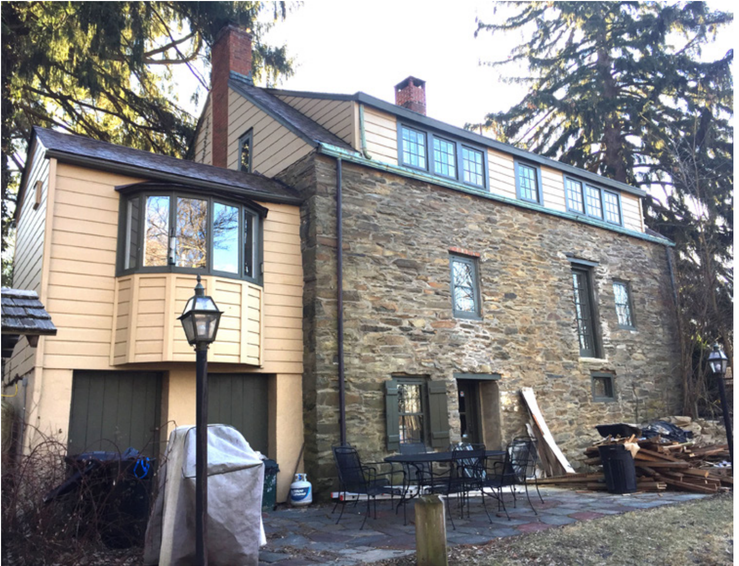
Fig.2: View of house from northwest. Photo by Neil Larson, 2018. The wood frame wing was added in the 1970s.
