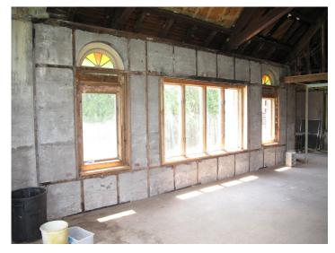
Fig.9: Great room, west wall showing loss of plaster, lath and studs embedded in concrete wall, 2021. Photo by Neil Larson.
