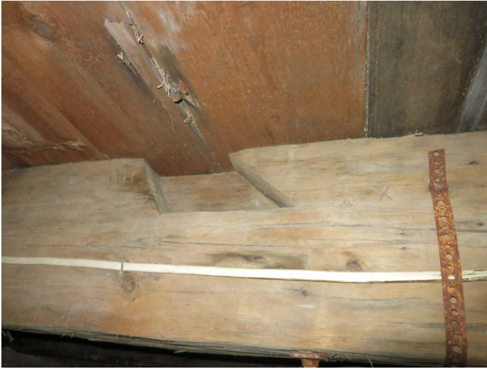
Photo 1. The open mortise that was formerly associated with the original stairs to the basement. This same detail is seen in another Montgomery County house on Reynolds Road, Town of Glen (Author photo, October 2020).
