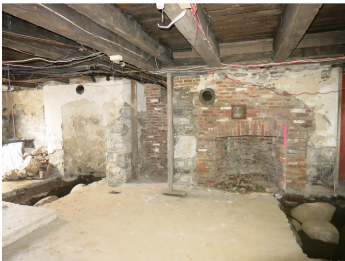
Photo 4. The east basement room of the 1773 portion of the house, showing the chimney supports and fireplace (Author photo, October 2020).
