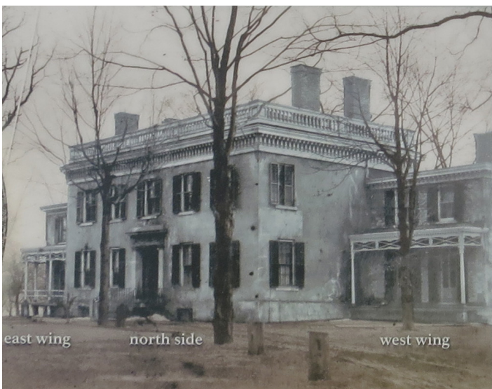
Figure 5. Undated photo, ca. 1880, showing the rooftop balustrade, stucco finish and other details added to the house in the 19th century.
