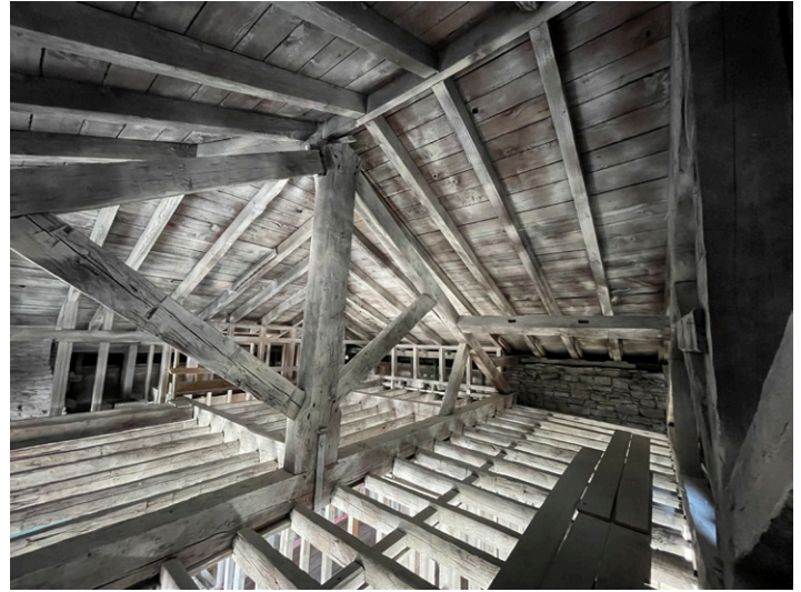
Photo 2. View of the roof framing after removal of second floor ceiling (unknown photographer, May 2023).
