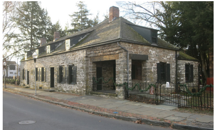
Photo 13b. Senate house today (photo taken in 2023; the house is currently under scaffolding).
