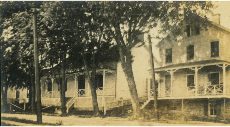
Photo 14. Bogardus House, on the corner of Washington Ave. and North Front St., on the west side of Washington Ave. Razed.
