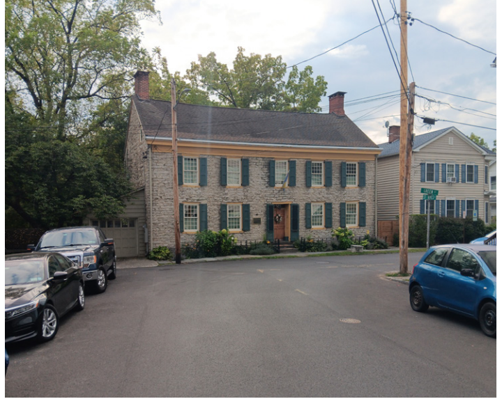
Photo 8b. 7 Green Street. The Cornelius van Buren house today (2025).
