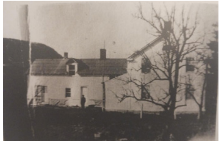
Figure 9. Side view of the Martin house, showing the ell, which may have been the original house. The Helderberg escarpment can be seen in the background, at left (Collection of Tim Albright).
